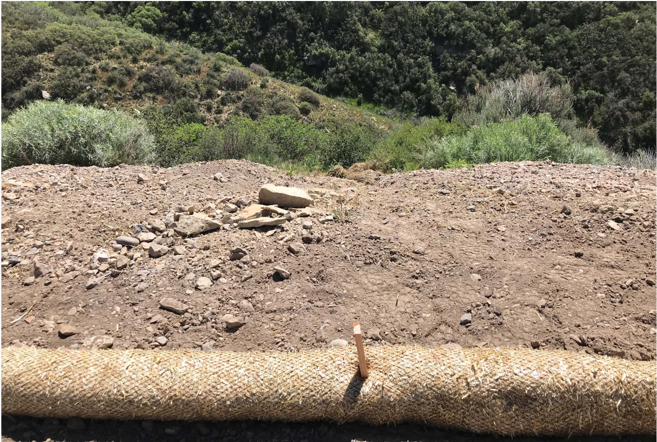
Area was repaired and new waddles were installed for sediment control.
