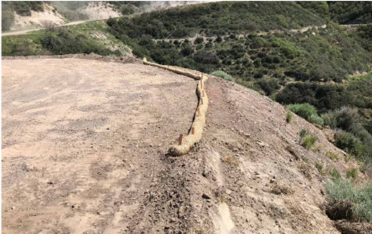
Area was repaired and new waddles were installed for sediment control.
