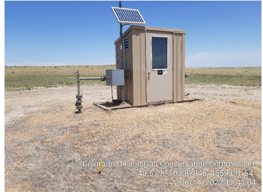
Photo 4 – Gas Injection Meter House
