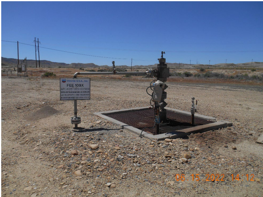
Injection wellhead.
