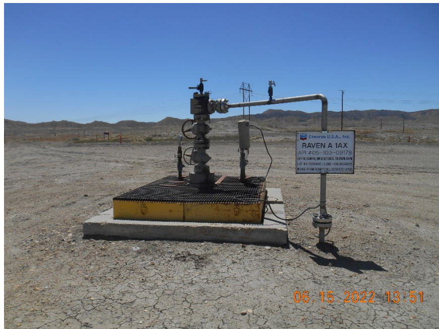
Injection wellhead
