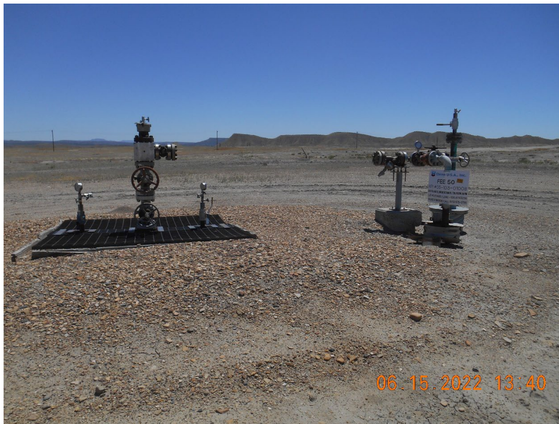
Injection wellhead. Temporarily Abandoned
