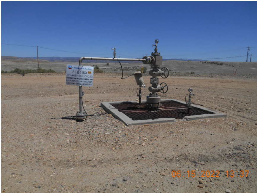
Injection wellhead
