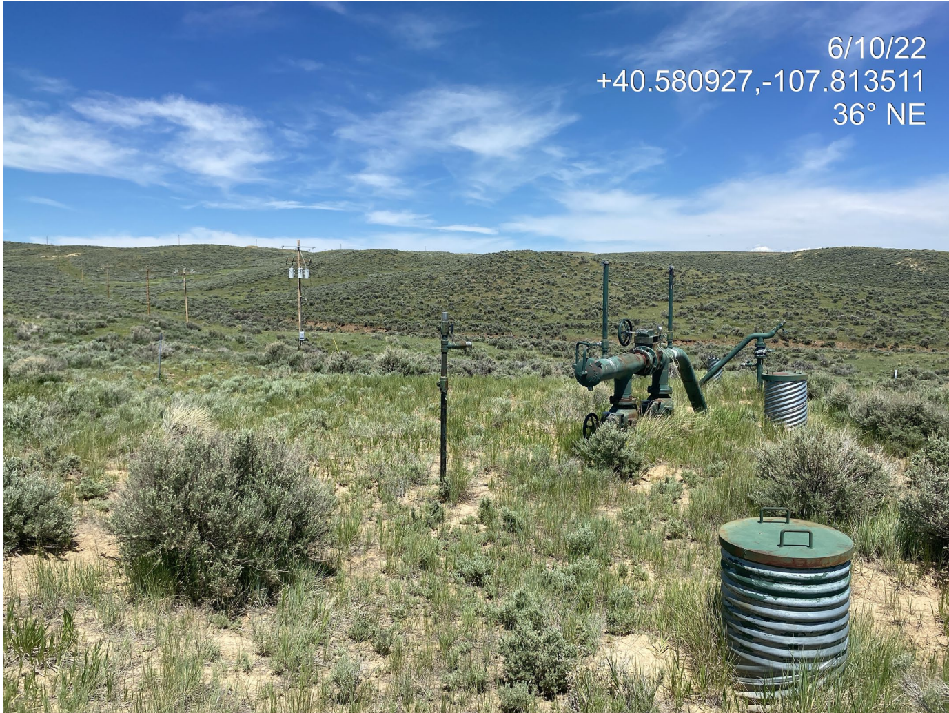
Photo 3. Photo taken from the south of the Location shows risers, pipes and power lines which must be removed for final reclamation per Rule 1004.a.
