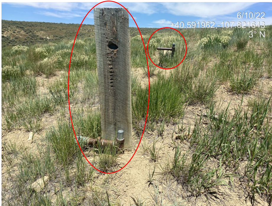
Photo 4. Photo taken from the south of the Location shows pipe equipment and a wooden post remaining on Location which must be removed per Rule 1004.a.
