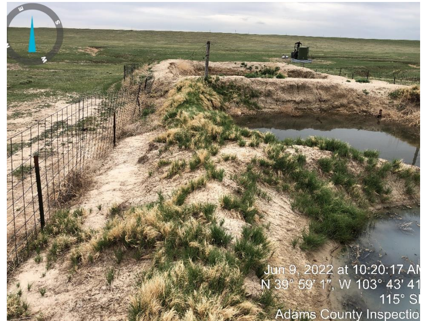
Photo #6 produced water pit 1 berm.
