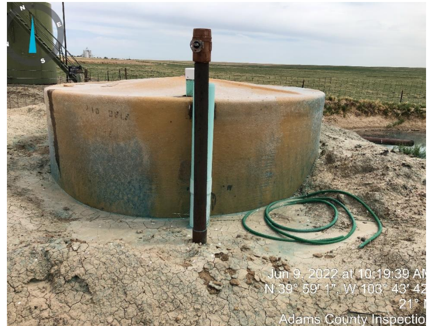
Photo #2 Produced water tank.
