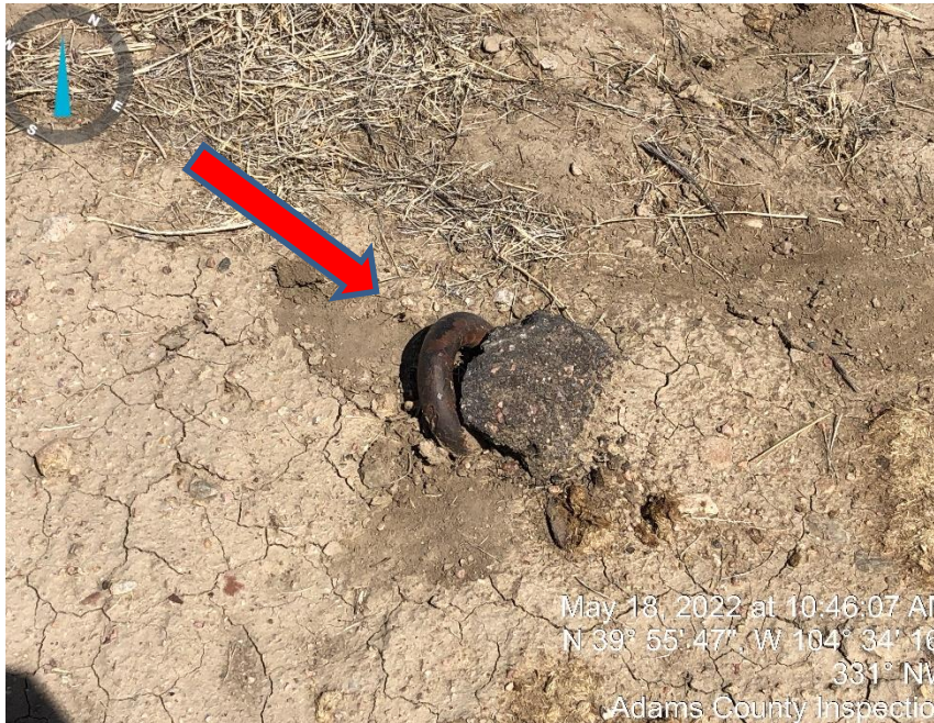
Photo #9 Unmarked guide line anchor.
