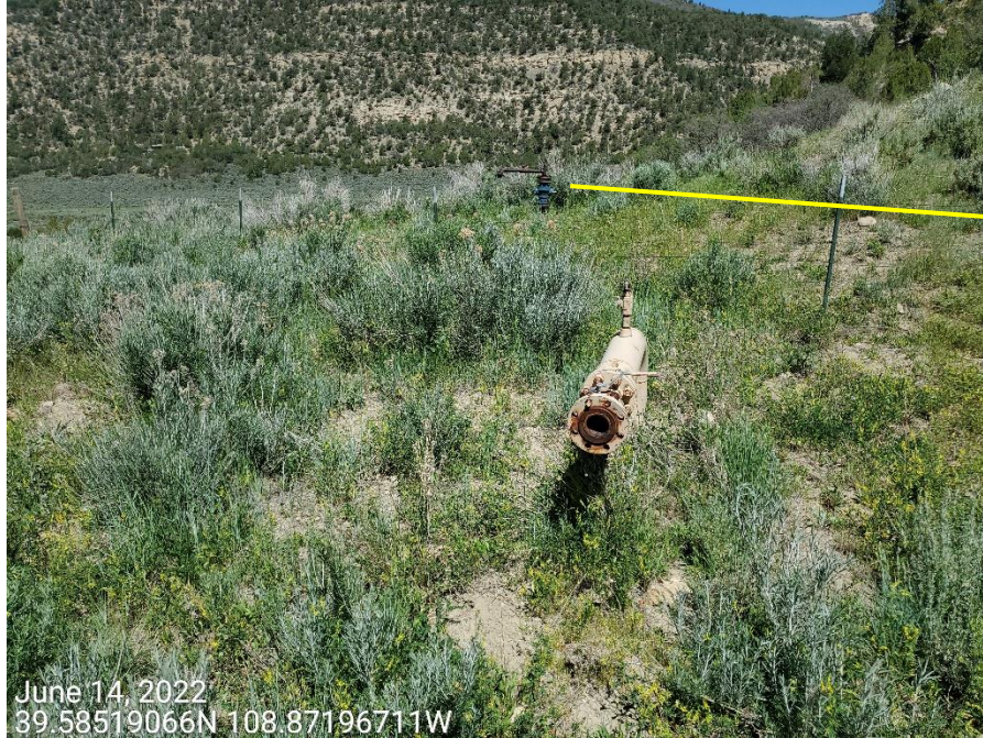
Photo 2: Photos taken from the North end of the Location. Photo shows piper risers / surface equipment remaining on the Locaiton. Equipment requires removal pursuant to Rule 1004.a
