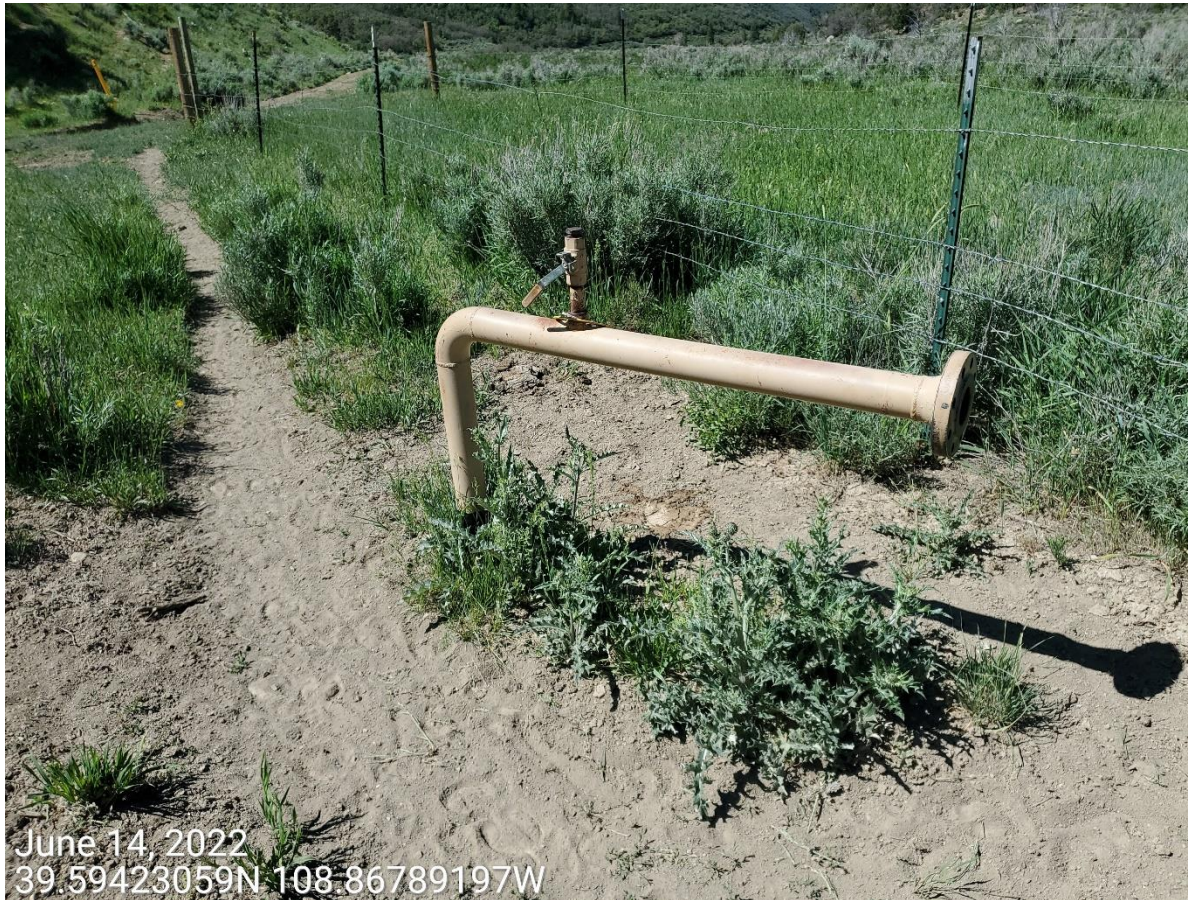
Photo 3: Photo shows riser equipment remaining on the Location; riser/surface equipment requires removal.
