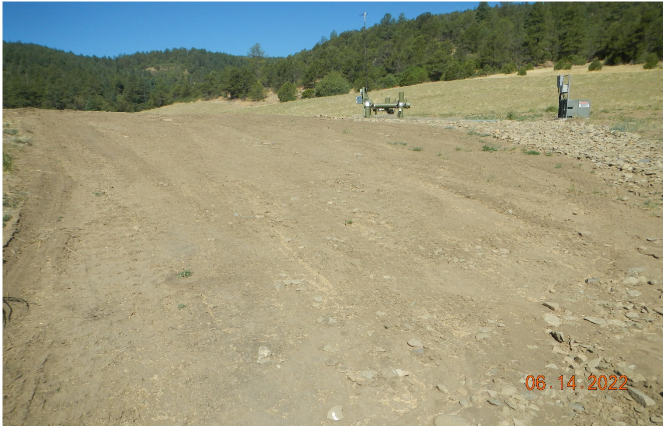
Photo 4. Facing toward the northeast side of the location. This area has been reseeded and rock rip/rap was installed in the erosion channel.
