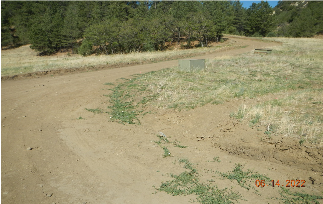
Photo 1. Facing west toward the access road ascending the hillside. The road has been graded. The culvert inlet cleaned out and repaired.
