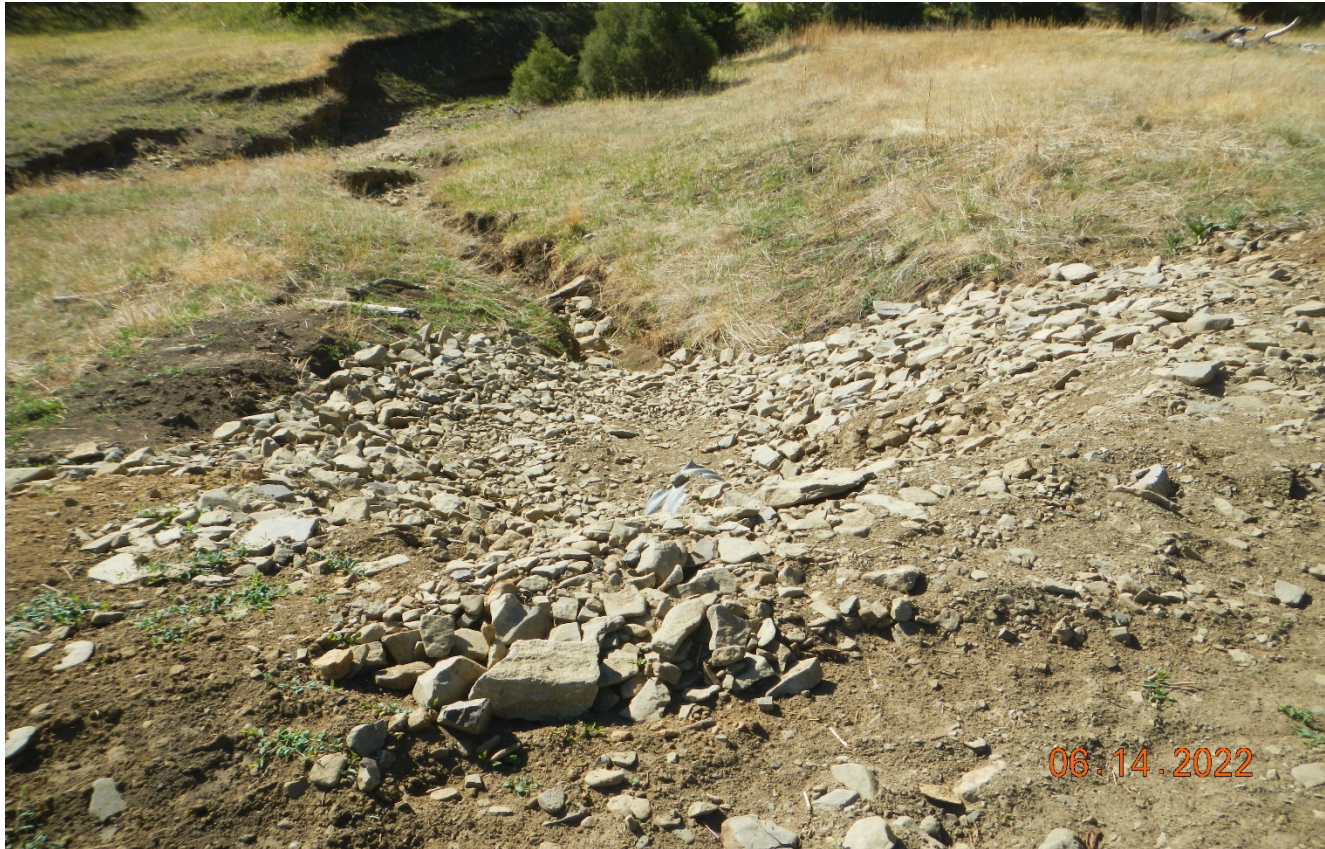
Photo 2. The culvert outlet has been repaired and rock rip/rap outlet protection has been installed.
