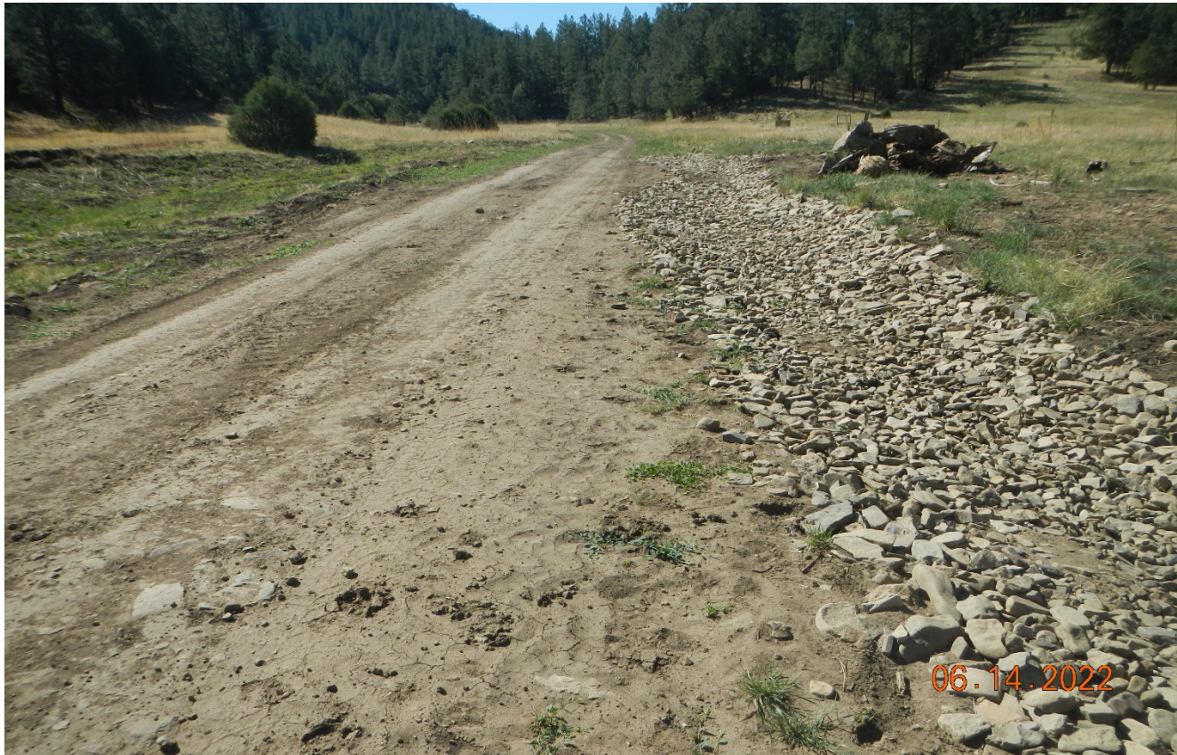
Photo 1. Facing southeast along the main road at the upper part of Lorencito Canyon. The erosion ins this area has been repaired. The culvert was removed and remains on the road side which needs to be removed.
