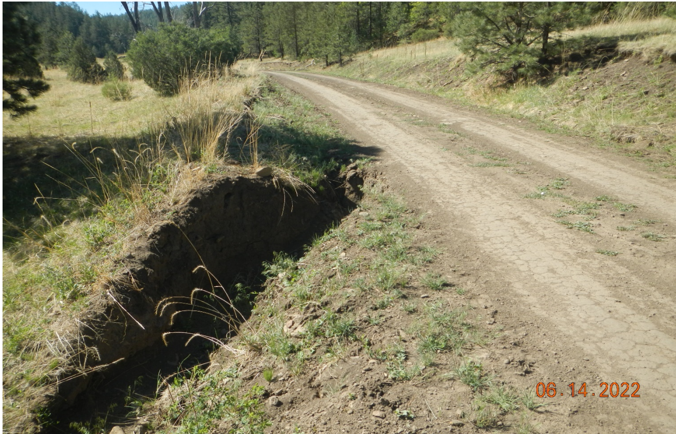
Photo 3. There is an erosion gully along the road that needs to be repaired and stabilized. Previous corrective action was not completed.
