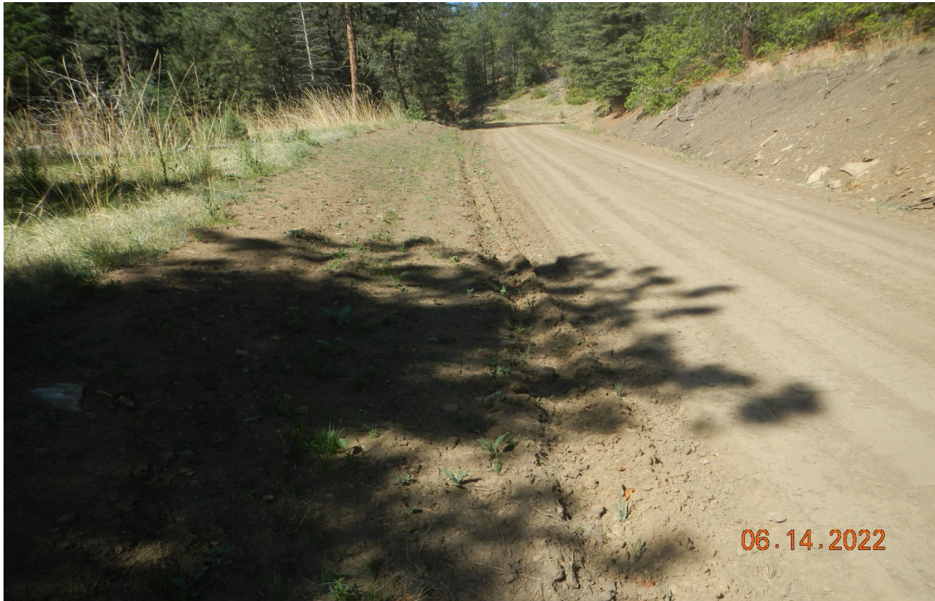
Photo 5. There was grading performed along the road. The disturbance along the side of the road needs to be seeded and reclaimed. Previous corrective action not completed.
