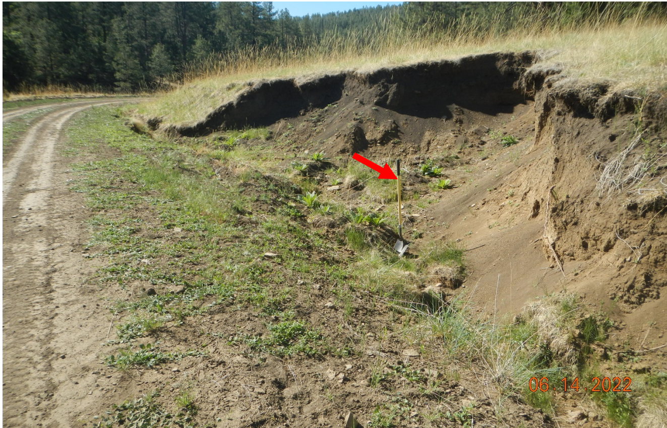
Photo 4. The side of the road is eroded and not stabilized at Lat/Long:36.99952,-104.83425. Erosion head cutting is continuing to occur further back. This area needs to be repaired and stabilized. Previous corrective action not completed. Red arrow points to 4.5 ft. shovel.
