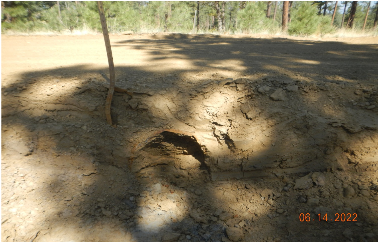
Photo 7. View of culvert from the previous photo which is full of sediment.
