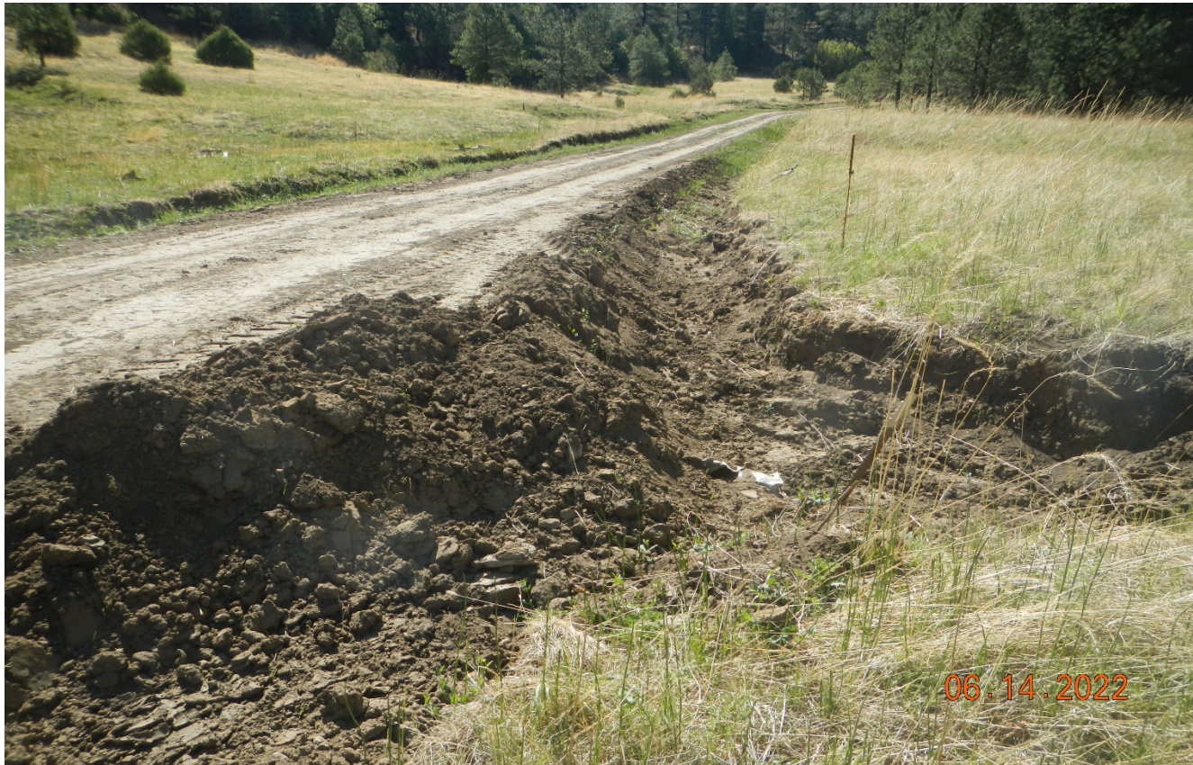
Photo 2. This culvert inlet was cleaned out however, the culvert is full of sediment which still needs to be cleaned out. Lat/Long:37.00581,-104.83861. Previous corrective action was not completed.
