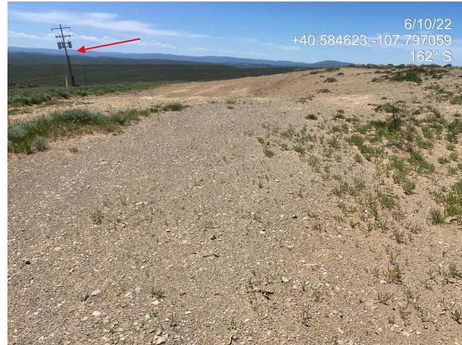
Photo 3. Photo taken from the northeast of the Location shows the access road, which must be reclaimed. Note also the power line remaining just off Location which must be removed and reclaimed.
