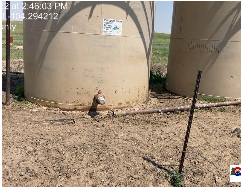
Pic 7 Previous leak from tank has been plugged
