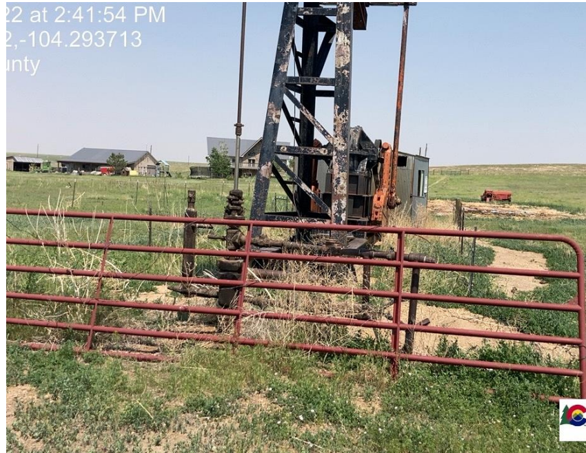
Pic 1 wellhead / pumpjack, weeds unmanaged, fence needs repair
