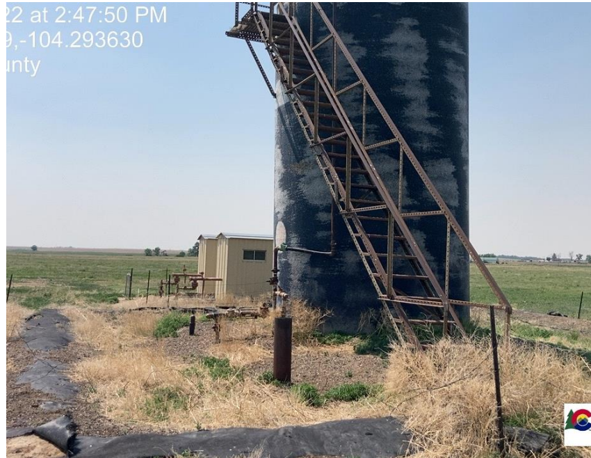
Pic 9 fiberglass tank berms are not adequate
