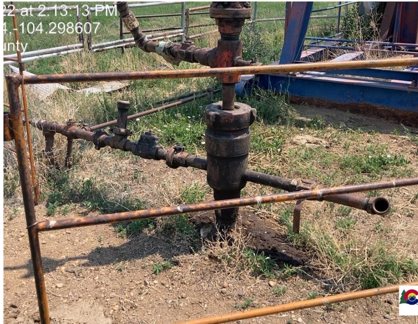
Pic 1 wellhead, bradenhead is not plumbed to surface, stained soil, weeds unmanaged
