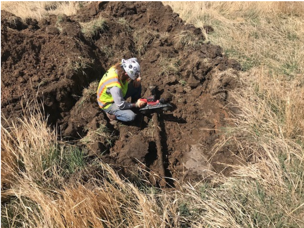
#6 – Cutting Flowline Prior to Pulling It Out
