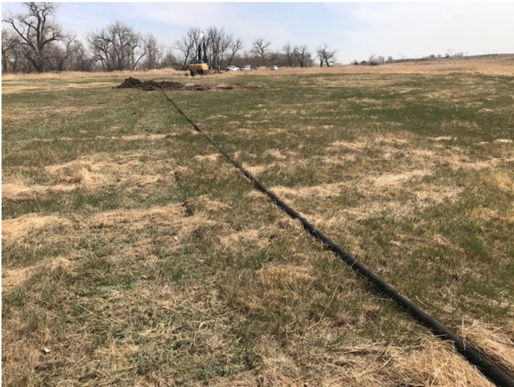
#8 – Pulled Flowline Allows Inspection
