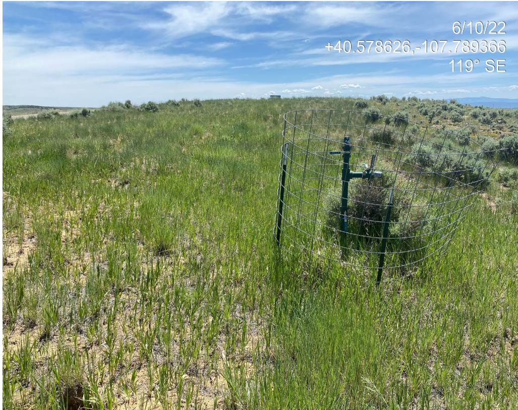
Photo 9. Photos taken from west of the Location across the road shows a pipeline riser which must be removed for final reclamation. Pipeline signage reads “Silver Stream Pipeline Company LLC” and “Pioneer Natural Resources USA Inc.”
