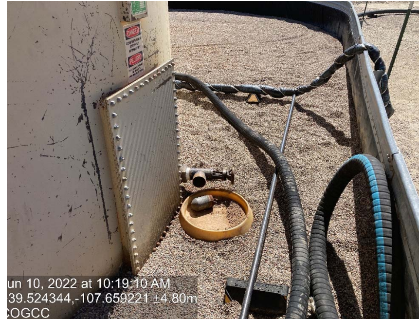
Valve missing cap/ plug
