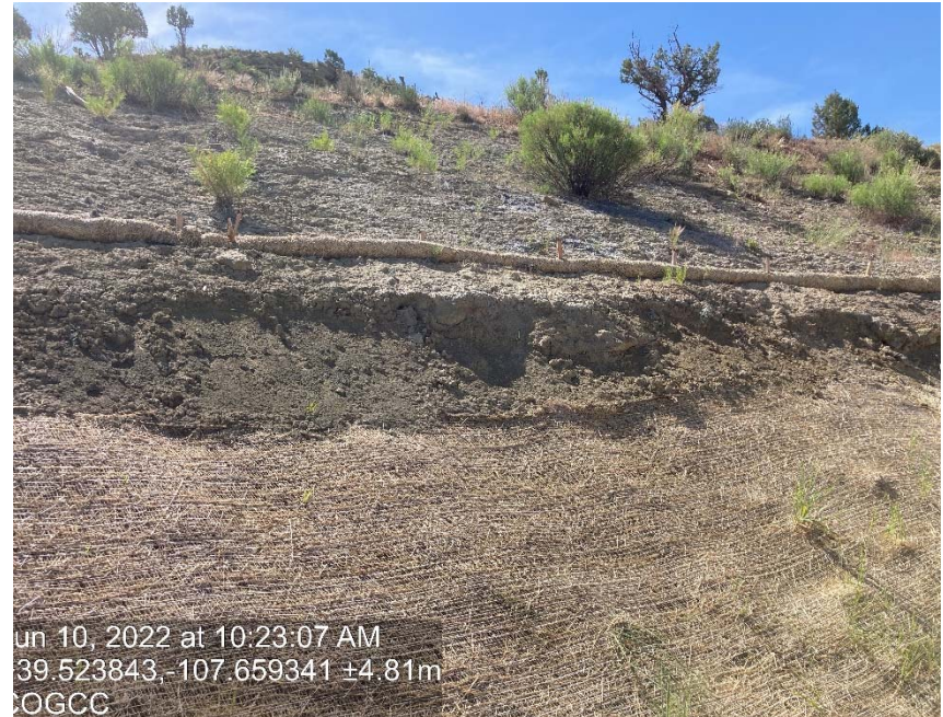
Cut slope erosion over blankets
