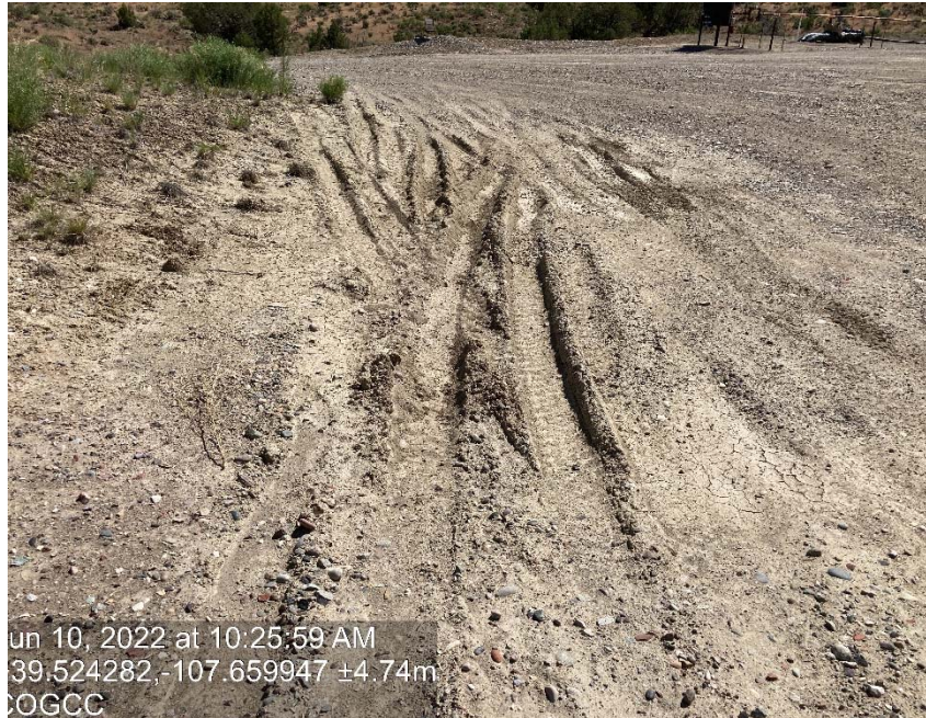
Lack of stabilization/ compaction/ degradation
