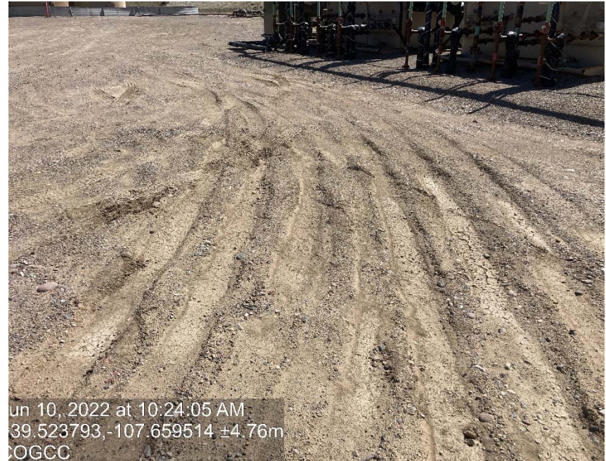
Lack of stabilization/ compaction/ degradation
