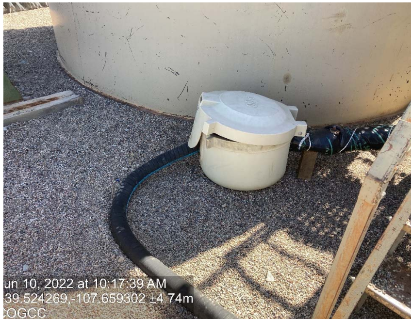
Valve missing cap/ plug
