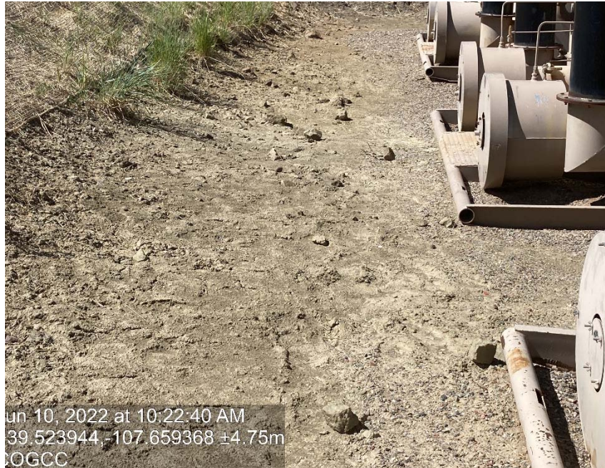
Evidence of cut slope erosion
