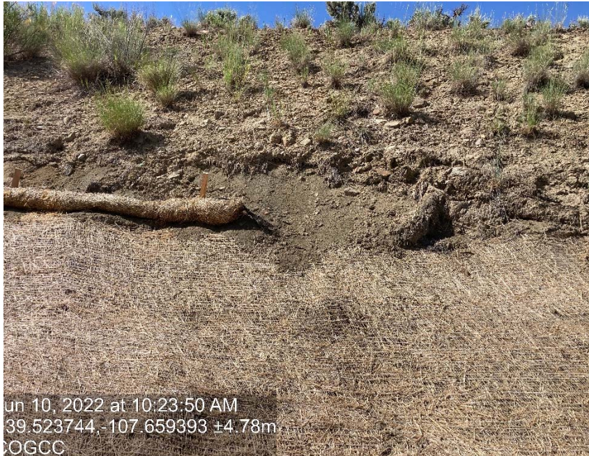
Cut slope erosion over blankets
