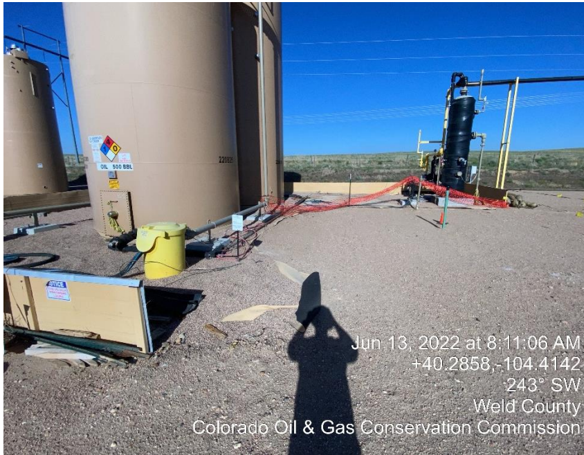
Photo #7 Containment wall needs repaired/ replaced
