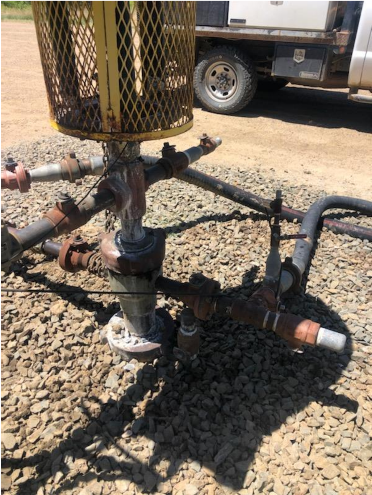
Installed appropriate fittings to allow bradenhead visual inspection as per Rule 419.a.(1),
