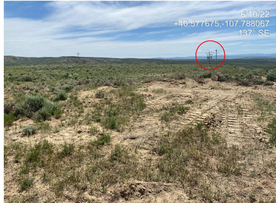
**Photo 2.** Photo taken from the northwest of the Location shows the reclaimed area being impacted by vehicle traffic. The power line (red circle) must be removed for final reclamation.
