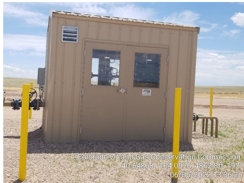
Photo 6 – Gas Lift Injection Meter House
