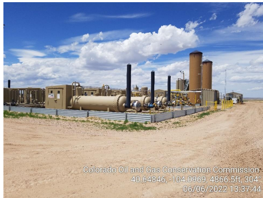
Photo 8 – Separators and ECDs
