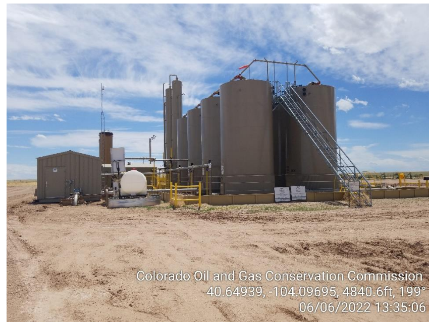
Photo 2 – Tank Battery and LACT
