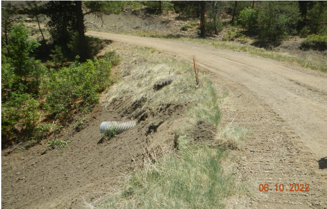
Photo 3. Further along the road at this drainage. The culvert has been repaired. It appears work is still in process for stabilization.
