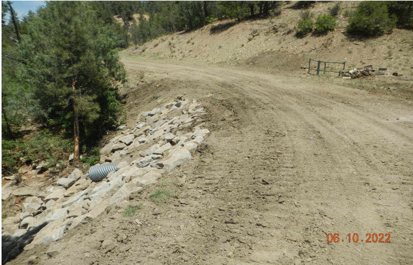
Photo 5. Facing west toward the well site. The road and culvert have been repaired at this drainage area.
