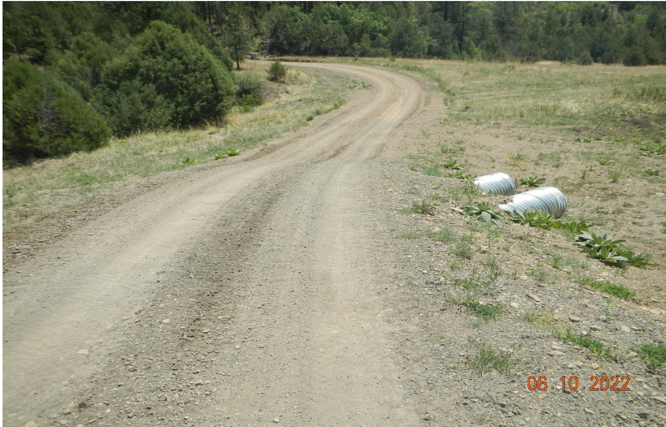
Photo 1. Facing east at the drainage crossing. This area was damage in the flood event where exposed pipe lines were observed. This area has been repaired.
