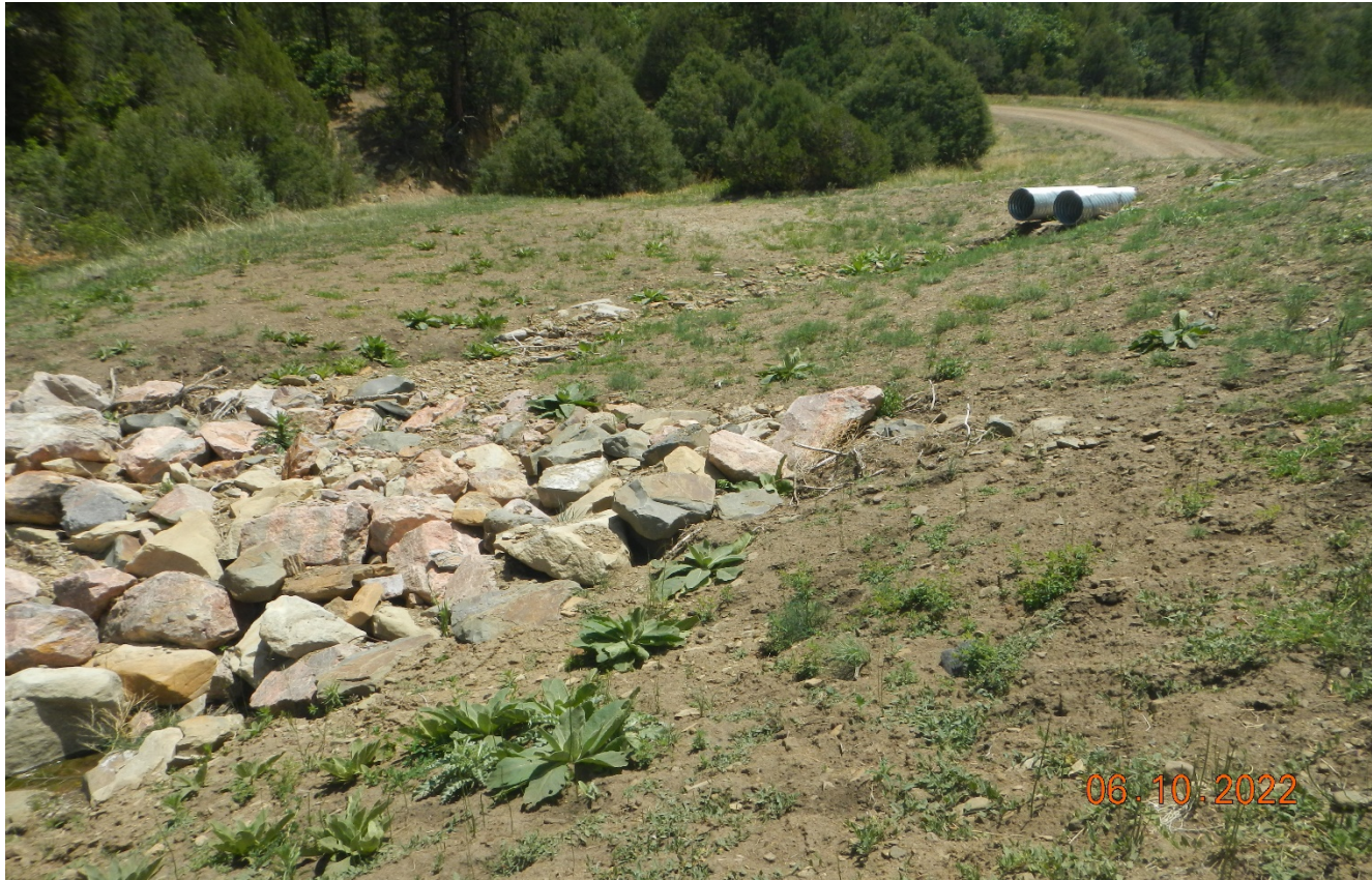
Photo 2. There is rock rip rap installed below the culvert outlets. Noxious weeds are beginning to sprout up in this area and will need to be controlled.
