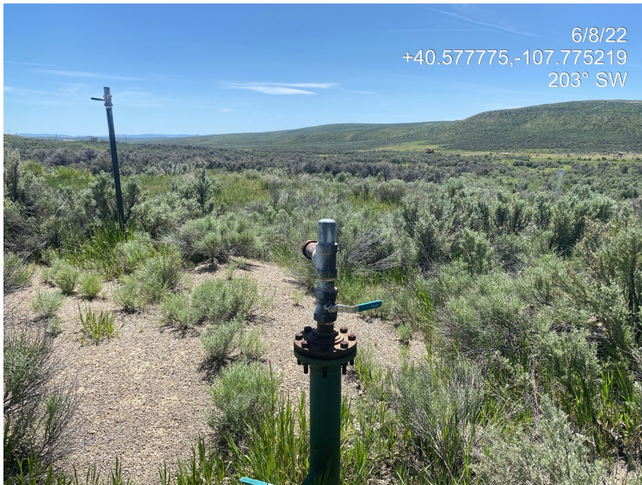
Photo 7. Photo taken from the west of the Location shows two risers which need to be removed for final reclamation.
