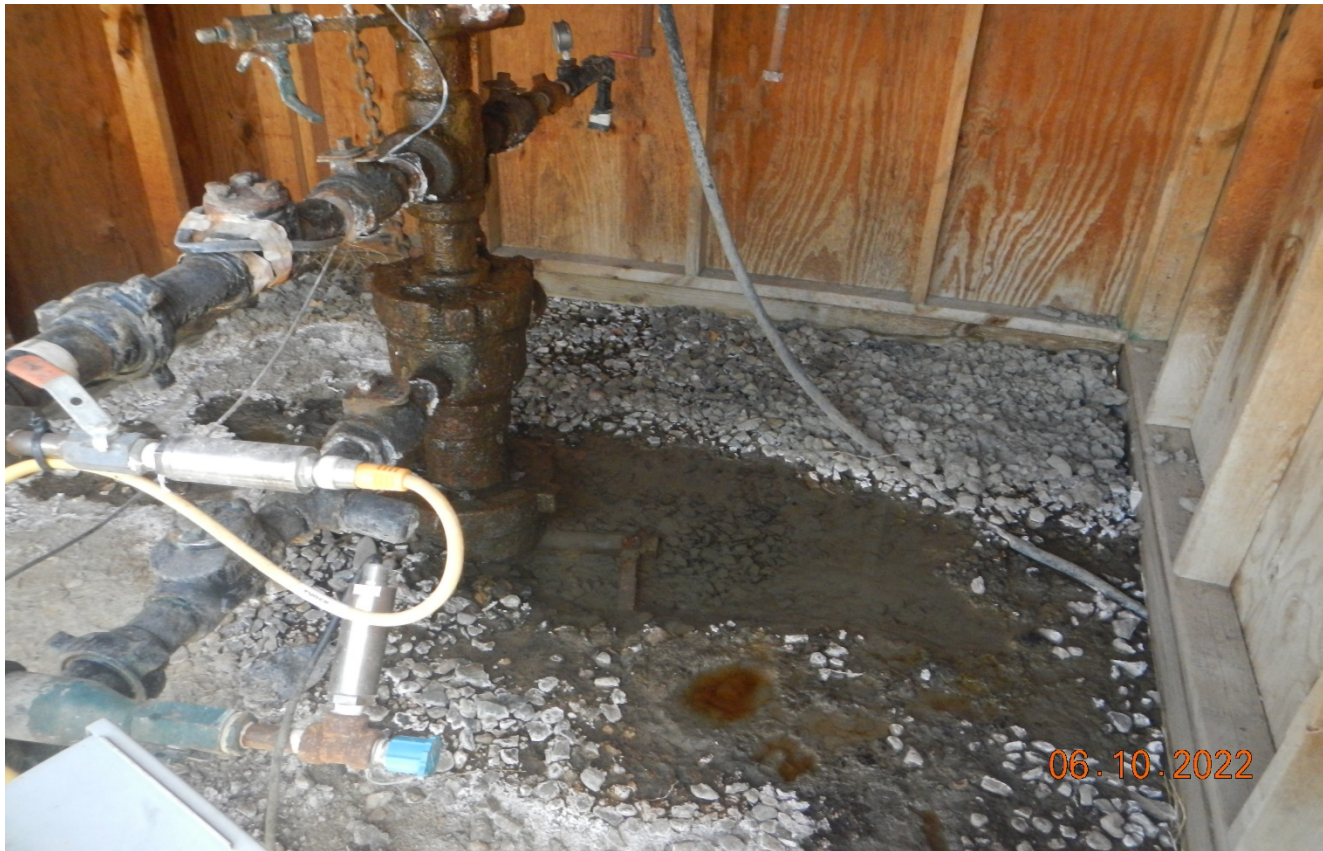
Photo 2. There is still a produced water leak at the wellhead that needs to be repaired.
