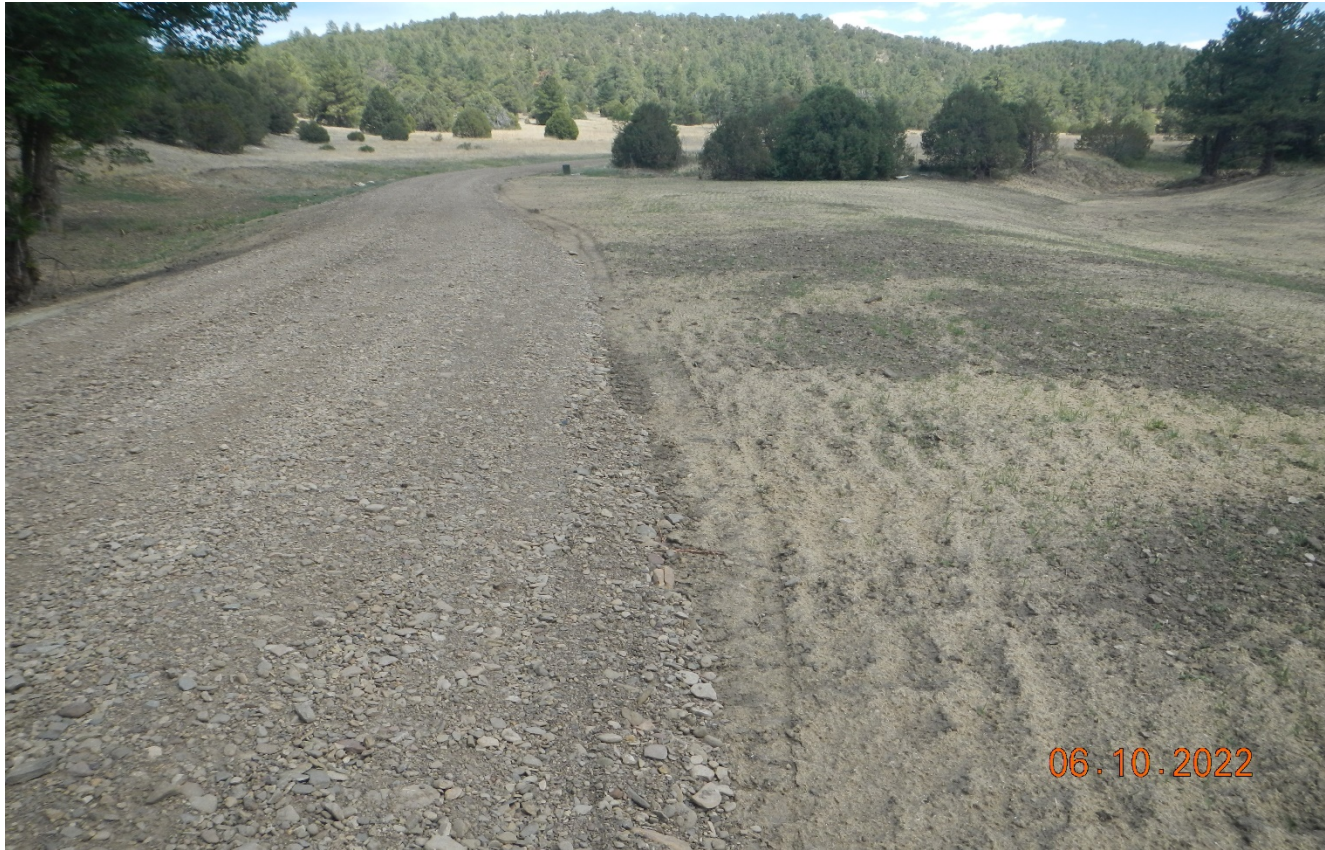
Photo 2. Facing southeast along the main access road. The road has been regraded and stabilized. Areas of disturbance are seeded and hydromulched.
