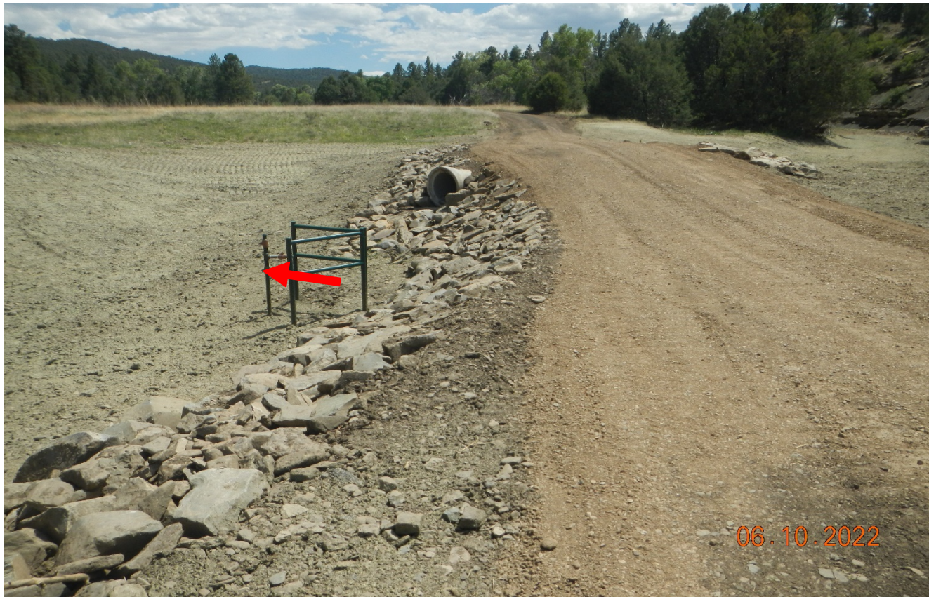
Photo 4. Facing south further along the main road. A new culvert has been installed and the crossing is repaired. A new flowline riser has been installed.
