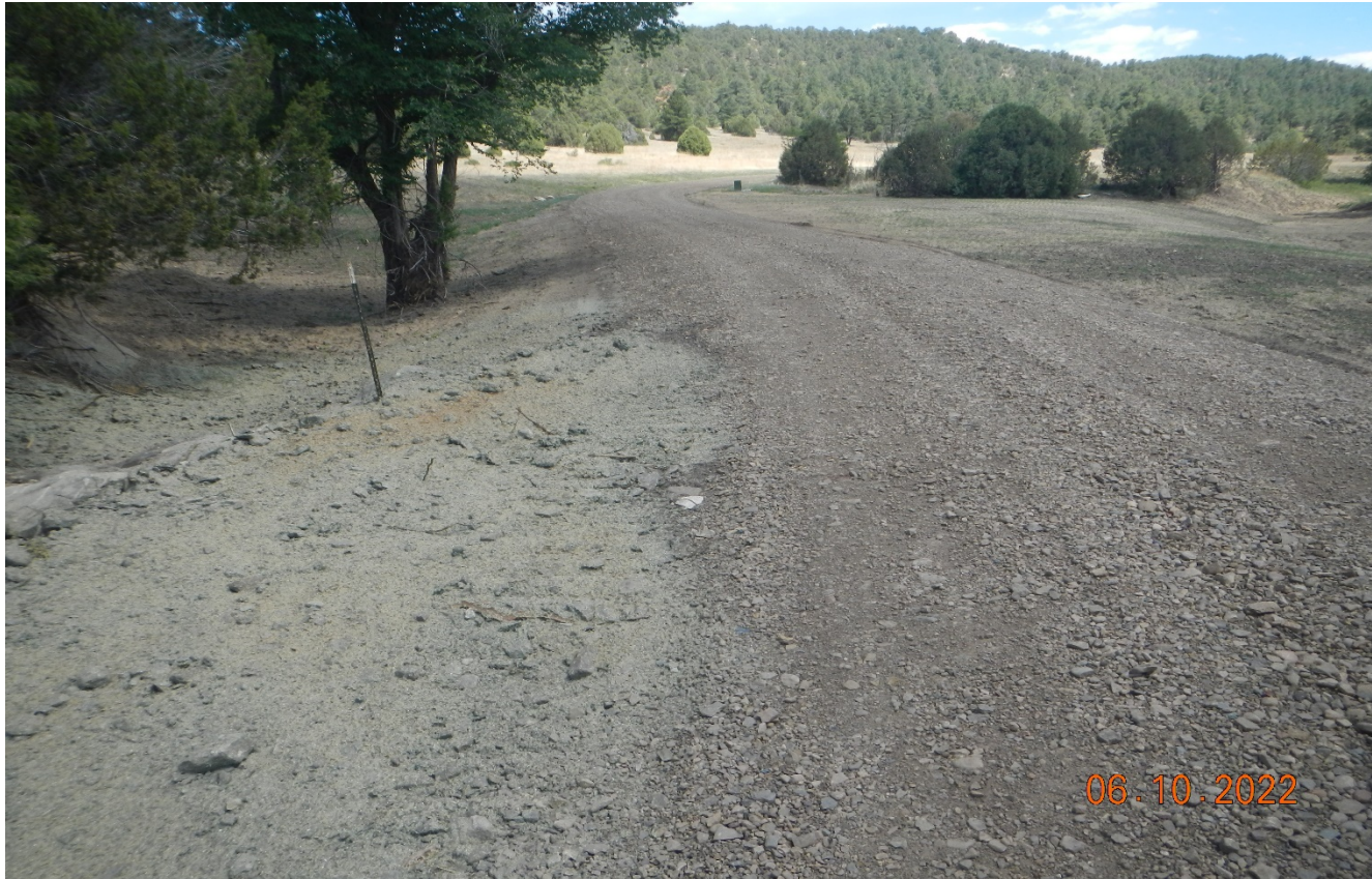
Photo 1. Facing southeast along the main access road. The road has been regraded and stabilized.
