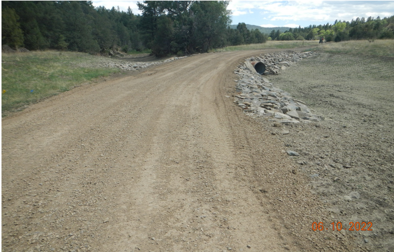
Photo 3. Facing south along the main road. A new culvert has been installed and the crossing is repaired.
