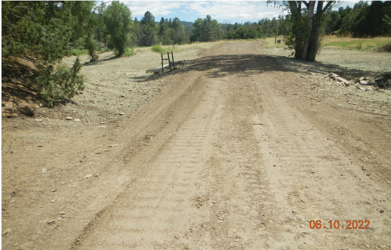
Photo 5. Facing south further along the main road. A new culvert has been installed and the crossing is repaired.
