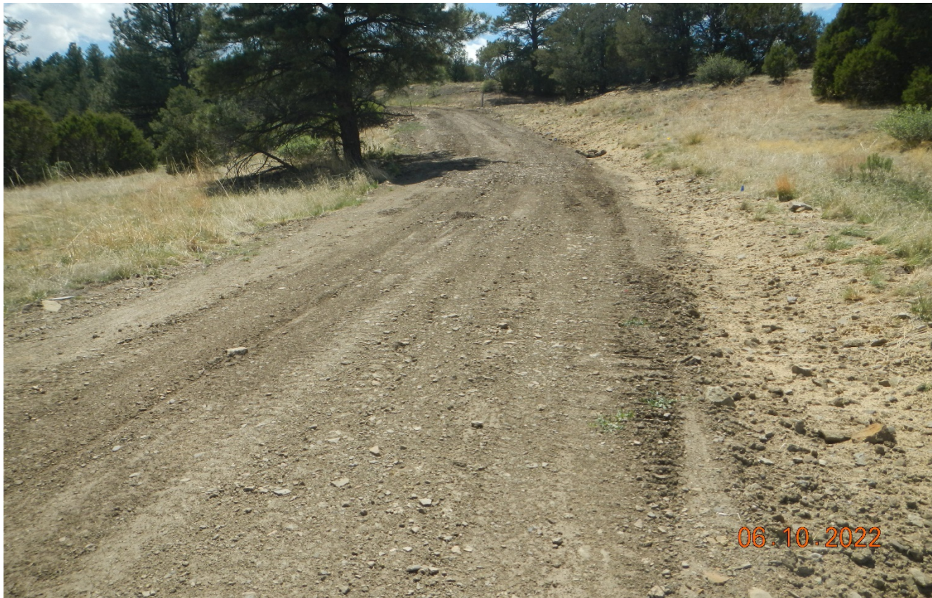
Photo 2. Facing southwest toward the access road. The erosion along the access road has been repaired.
