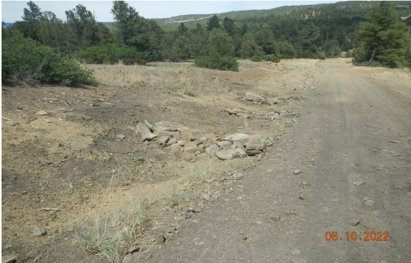
Photo 3. There are rock check dams installed along the road side.
