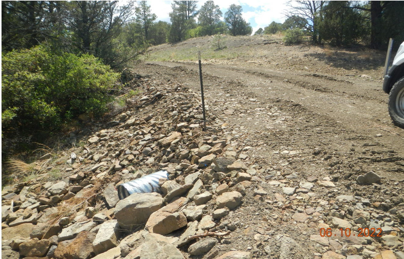
Photo 4. Further up the access road. A new culvert has been installed along the road to divert stormwater.
