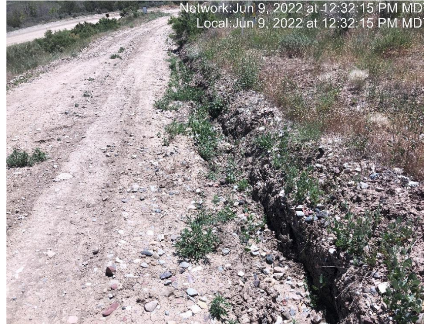
Photo #6878 Gully erosion occurring in access road ditch. Insufficient velocity checks in ditch.
