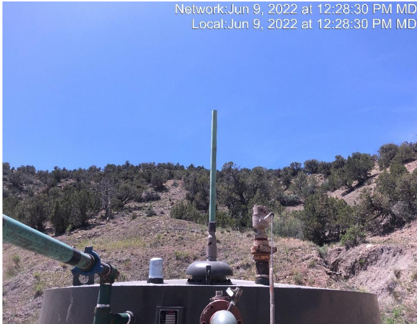
Photo #6869 Vent pipe on tank open ended.
