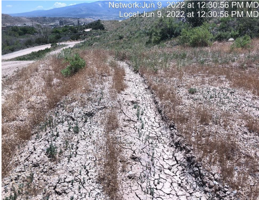
Photo #6872 Insufficient velocity checks in ditch.
