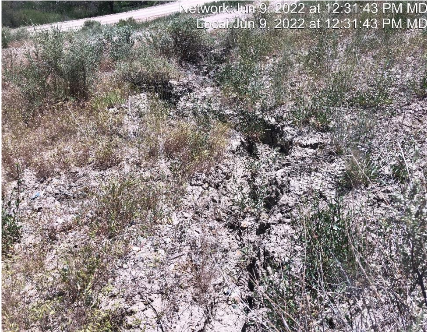
Photo #6875 Gully erosion occurring on cut slope.
