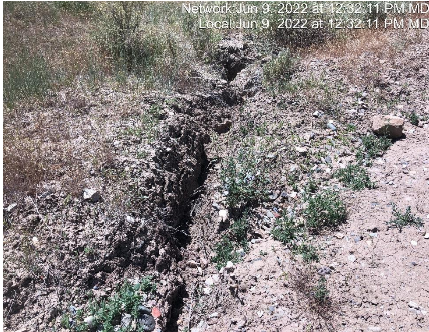
Photo #6877 Gully erosion occurring on cut slope.
