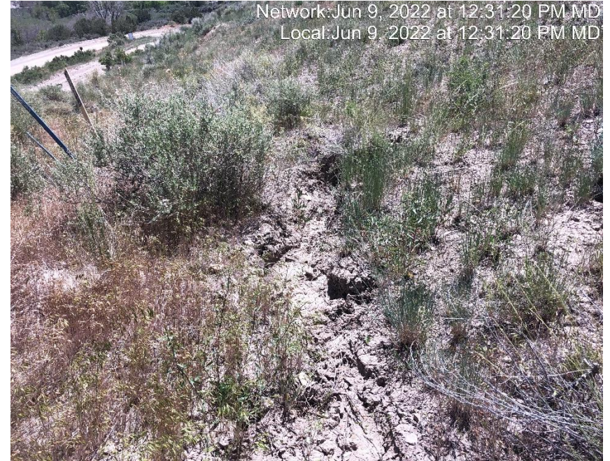
Photo #6873 Gully erosion occurring on cut slope.
