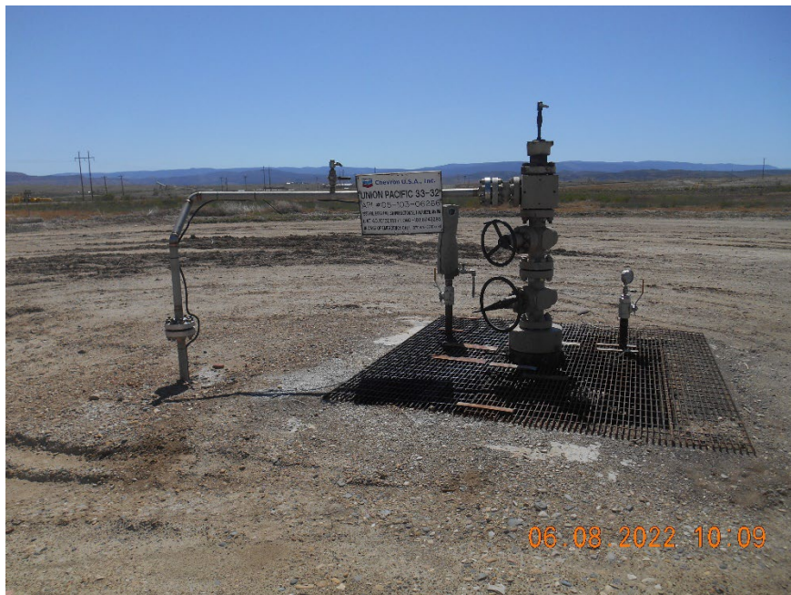
Injection wellhead.
