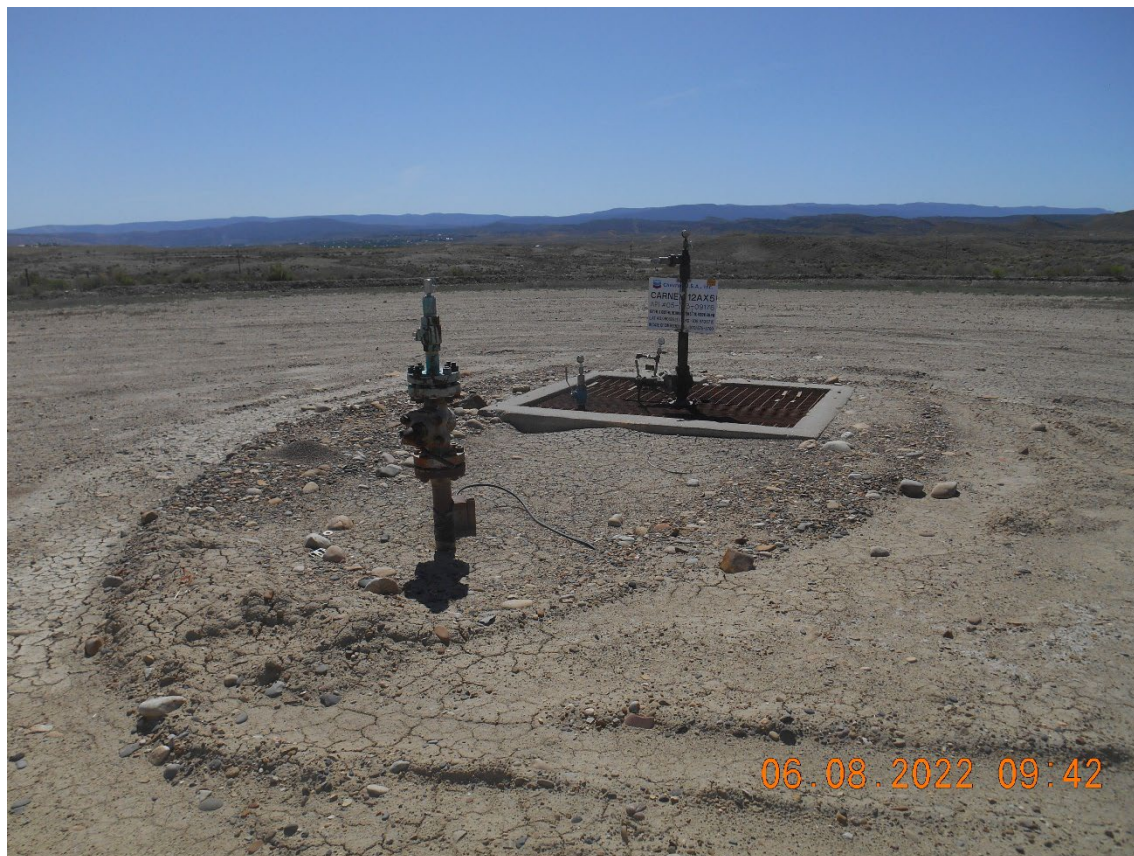
Injection wellhead (Temporarily Abandoned)
