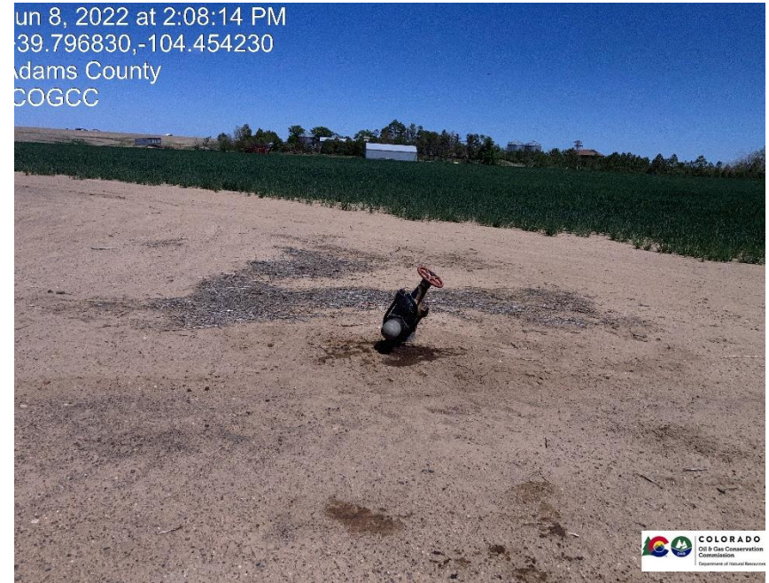
Pic 4 riser on location has mechanical issue / stained soil needs to be removed
