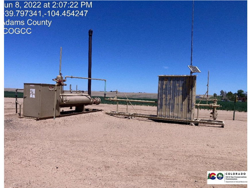
Pic 2 gas meter run, separator
