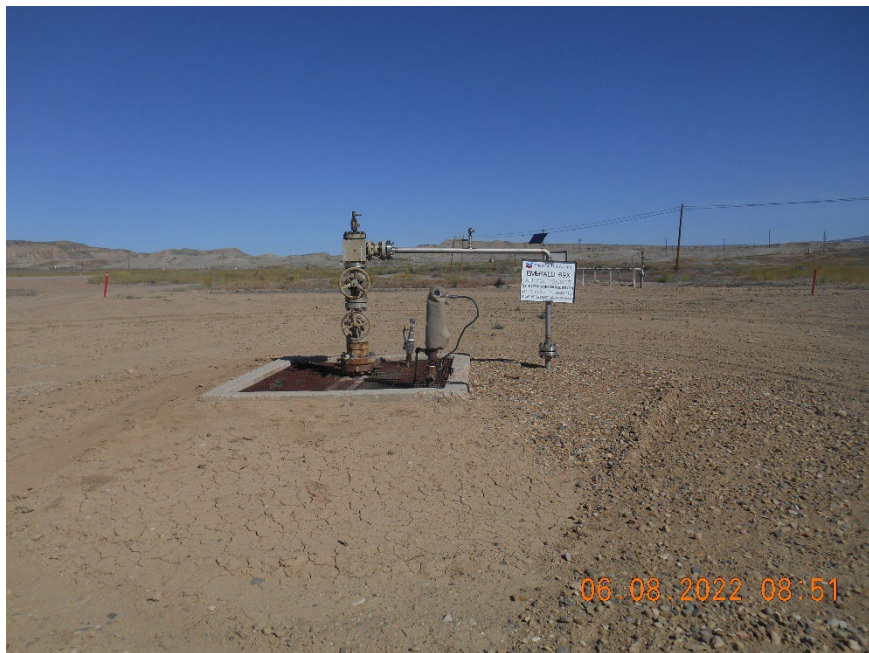
Injection wellhead
