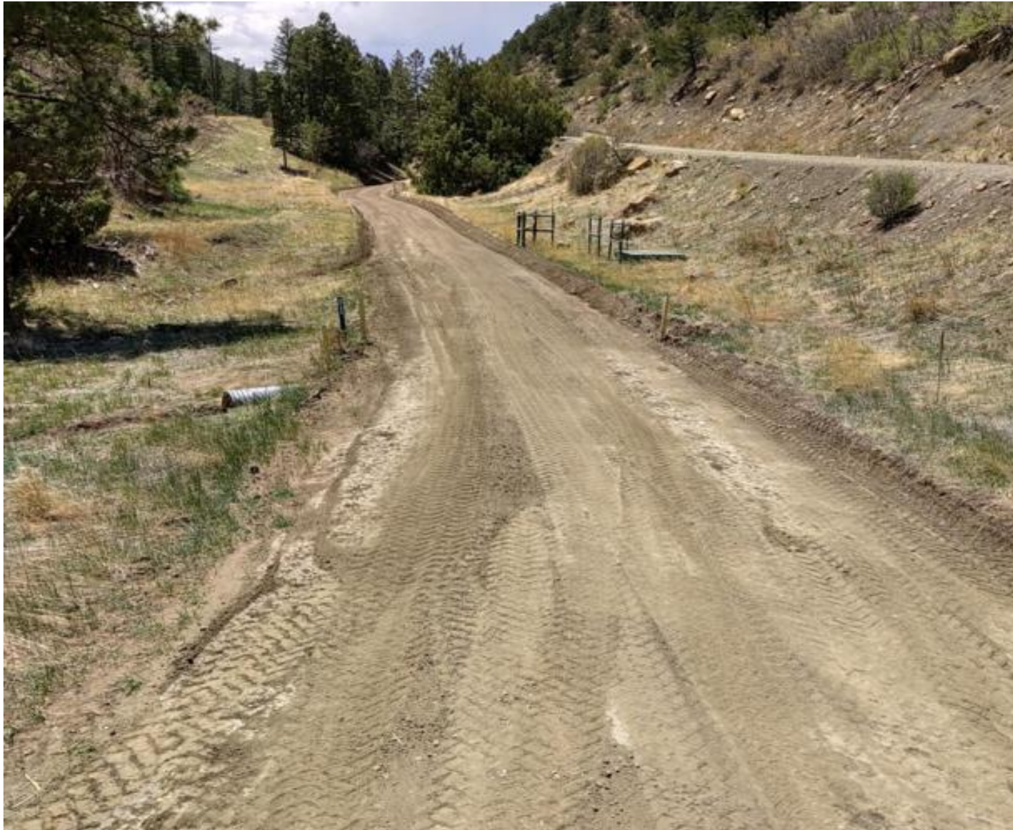
PHOTO 1: THE ROAD SURFACE HAS BEEN STABILIZED AND CROWNED TO CREATE SHEET FLOW AND ELIMINATE THE TIRE RUTS. THE BAR DITCH ALONG THE ENTIRE ACCESS WAS MODIFIED TO RECEIVE STORMWATER RUN OFF FROM THE ACCESS ROAD AND DIRECT RUN OFF TO THE CULVERT INLETS. VARIOUS WATER TURNOUTS WERE INSTALLED TO ALLOW STORMWATER TO DRAIN FROM THE ROADWAY SURFACE. CULVERT MAINTENANCE HAS BEEN PERFORMED ALONG THE ENTIRE ACCESS.
