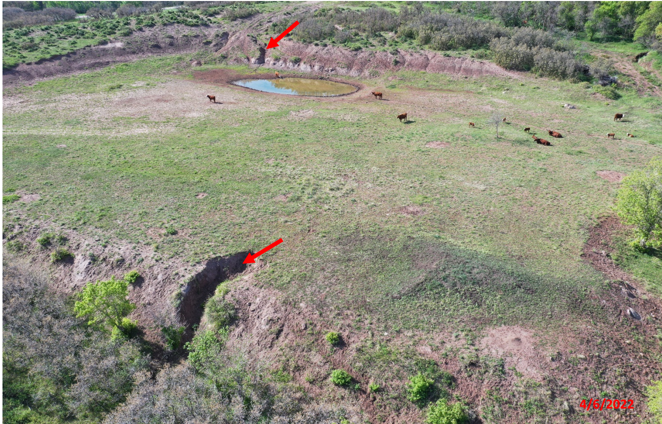
Photo 6. Facing southwest overlooking the location. There are multiple areas of significant gully erosion along the cut and fill slopes shown at red arrows.
