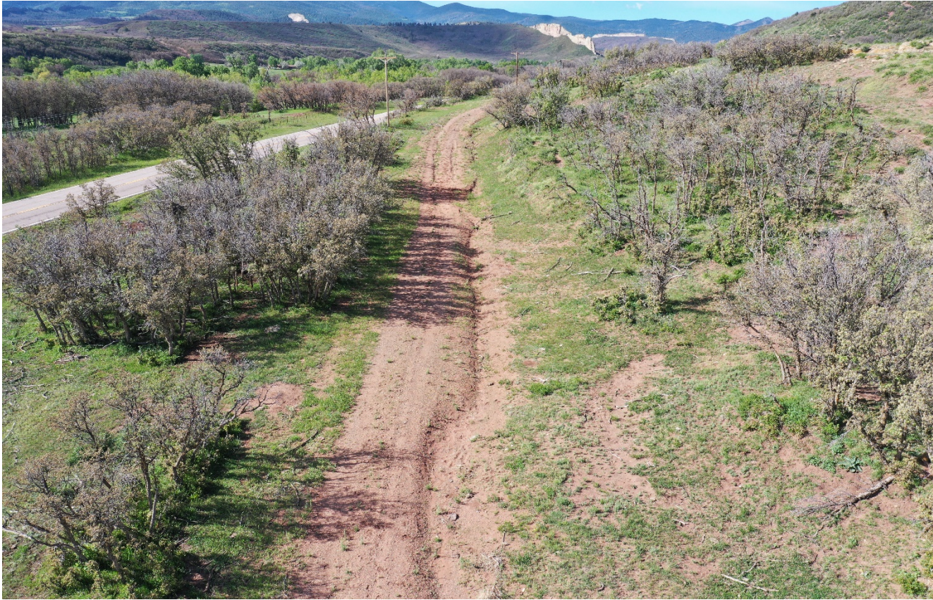
Photo 2. Drone aerial photo facing southwest along the access road. There is erosion occurring along the road which has not been repaired and stabilized.
