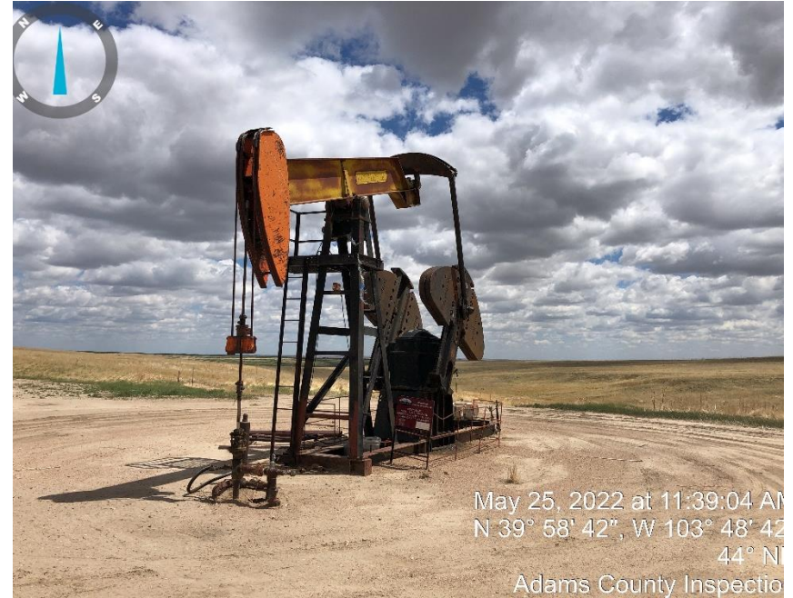
Photo #6 Pump Jack.
