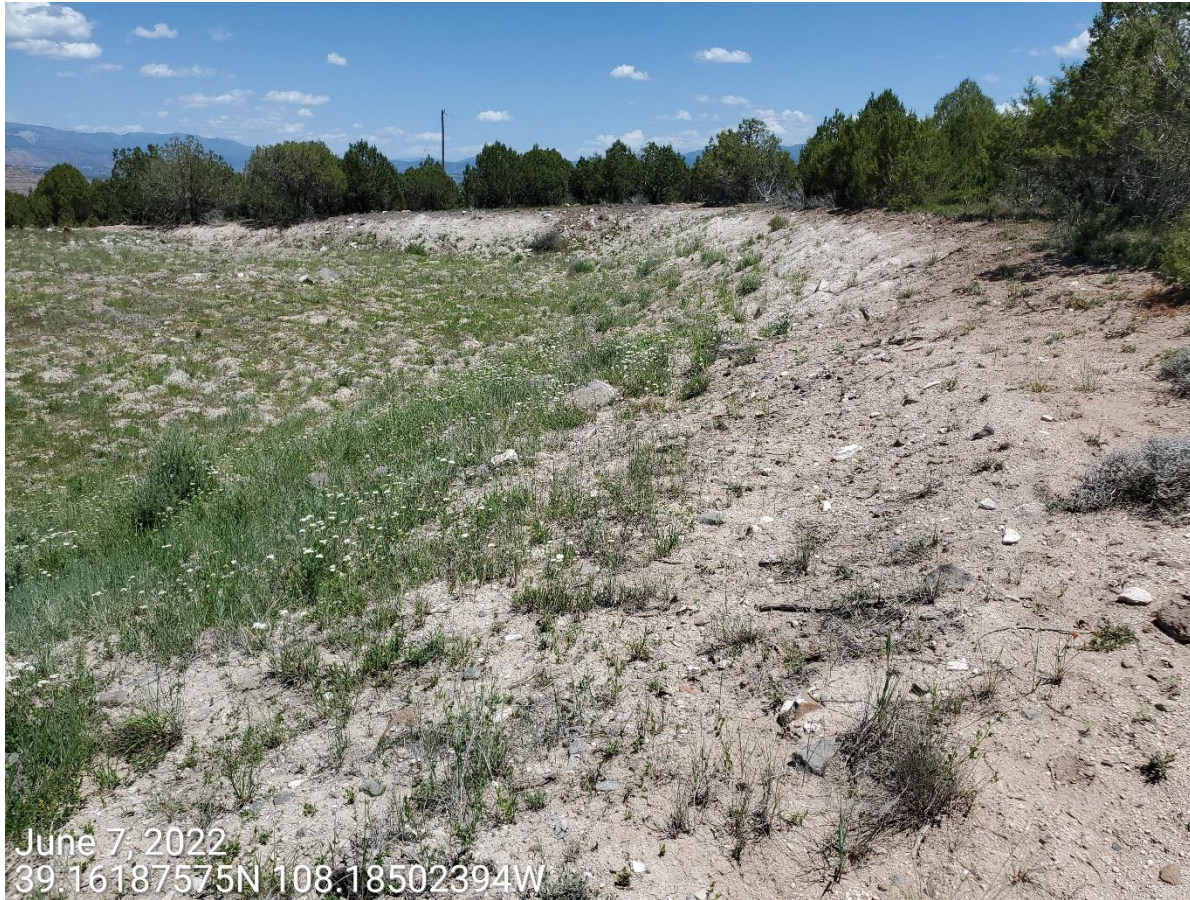
Photo 2: Photos show Location has not been recontoured/regraded; cut slopes evident. Reclamation of the Location has not been completed in accordance with 1004 requirements.
