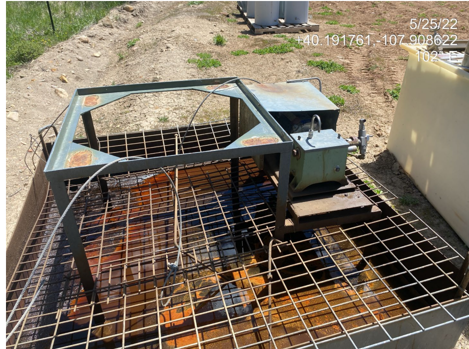
Photo 4. Photo taken from the west of the Location shows a secondary containment tank lacks control measures to allow for wildlife egress.
