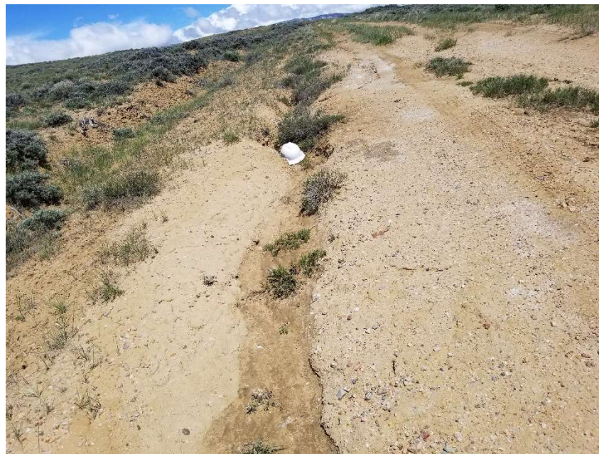
Photo 2. Erosion on access road.
