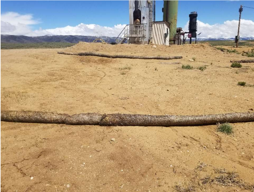
Photo 5. Sediment migration occurring under and through wattles.
