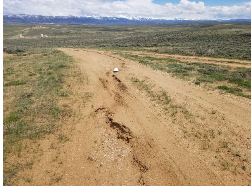
Photo 4. Erosion on access road. Hardhat for scale.
