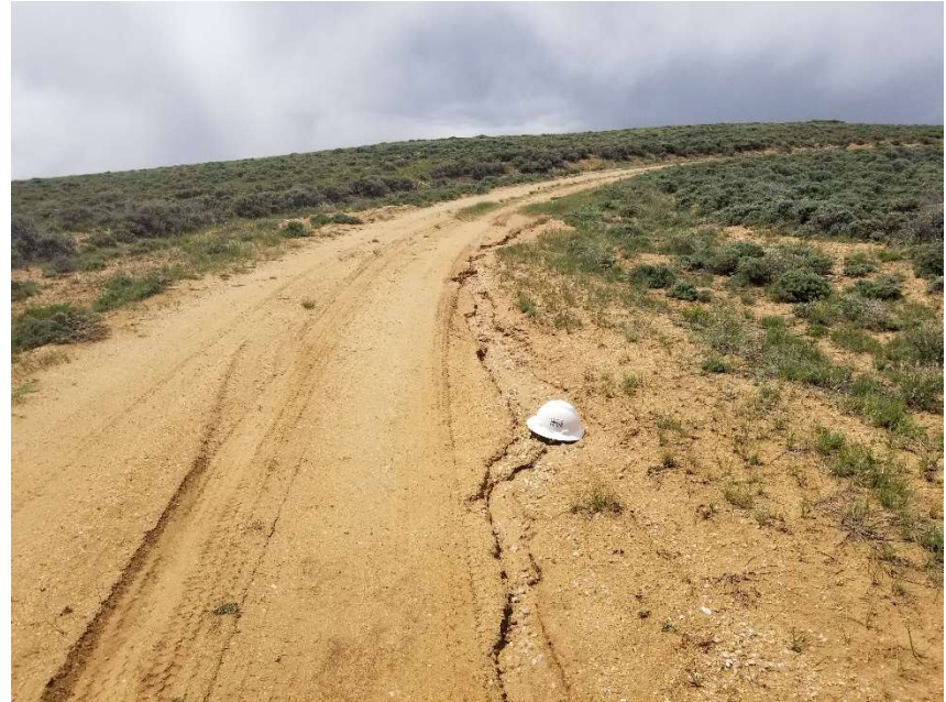
Photo 2. Erosion on access road. Hardhat for scale.
