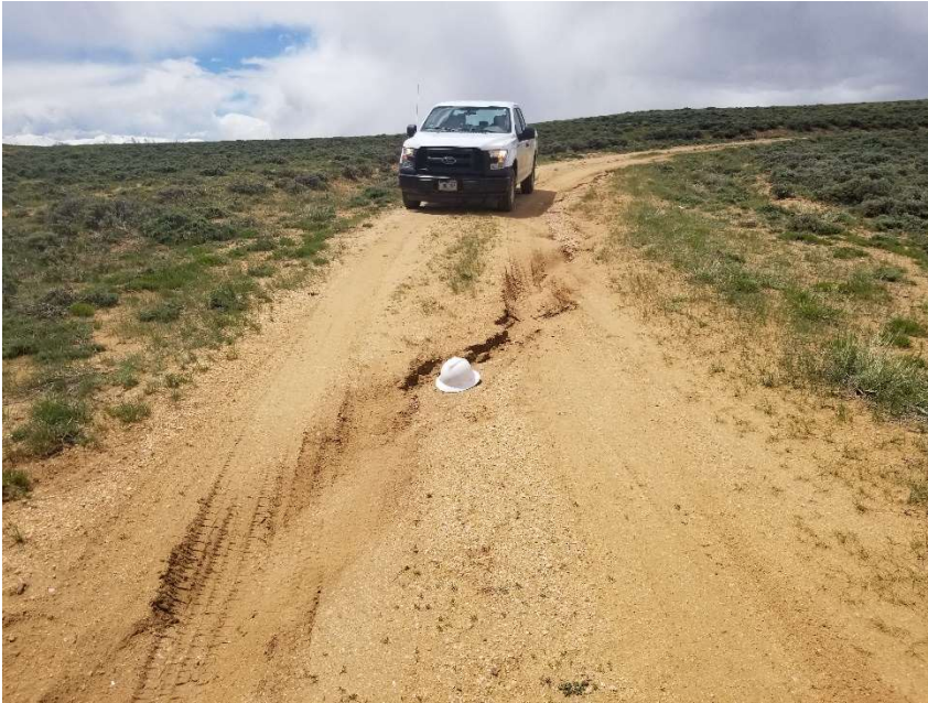
Photo 3. Erosion on access road. Hardhat for scale.
