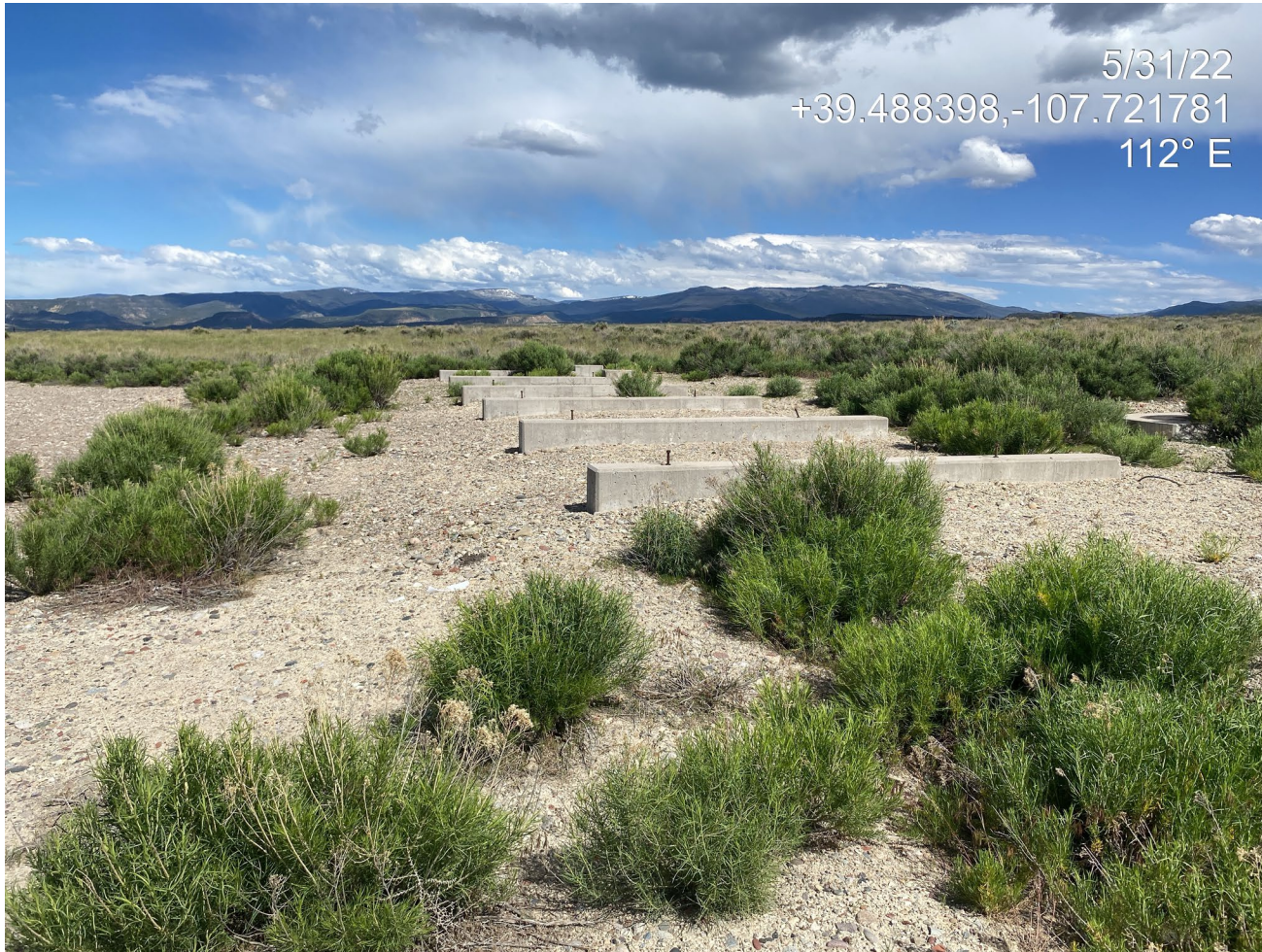
Photo 2. Photo taken from the south of the Location shows concrete forms no longer in use and adjacent areas requiring interim reclamation.
