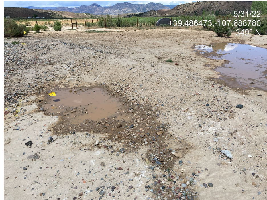
Photo 2. Photo taken from the east of the Location behind the separator shows the previously undermining berm is intact. Photo shows the view from the inside of the berm.
