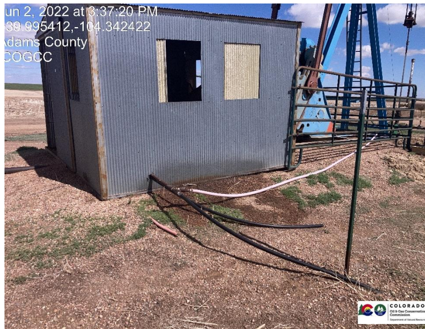
Pic 9 chemical tank leak, stained soil visible on outside of motor house, no containment used on chemical tank(s)
