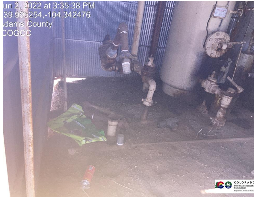
Pic 5 trash and stained soil in separator house
