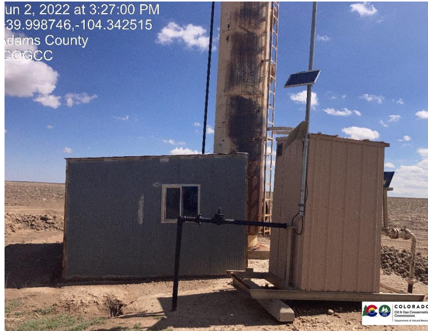
Pic 3 gas meter run, separator
