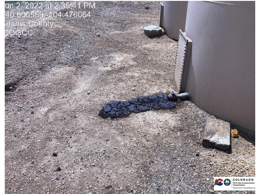
Pic 4 stained soil / mechanical issue back of tank
