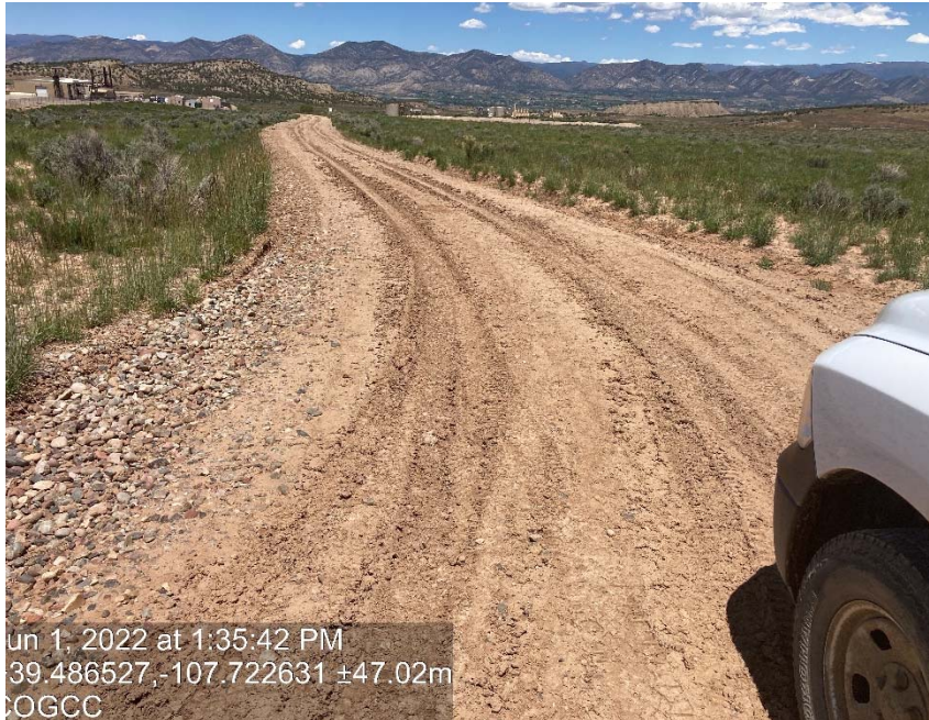
Lack of stabilization/ compaction
