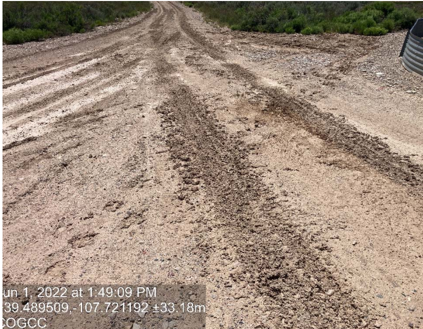
Lack of stabilization/ compaction
