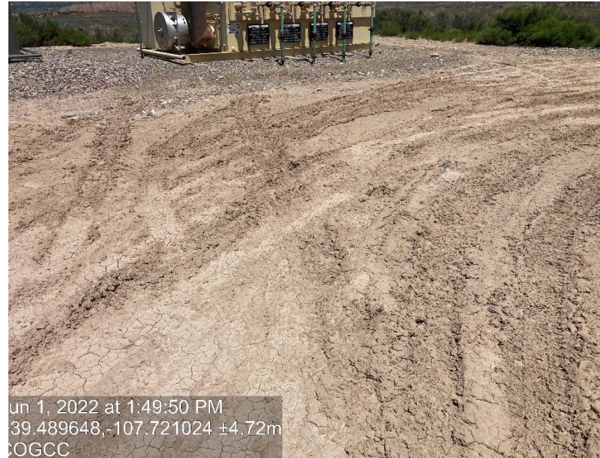
Lack of stabilization/ compaction
