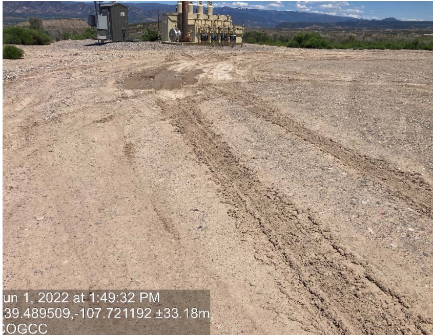
Lack of stabilization/ compaction
