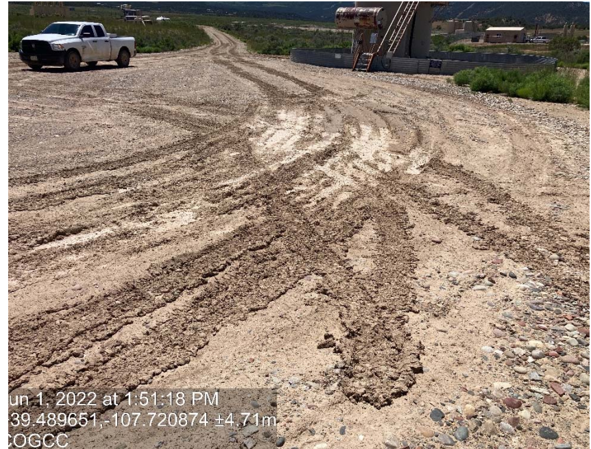
Lack of stabilization/ compaction
