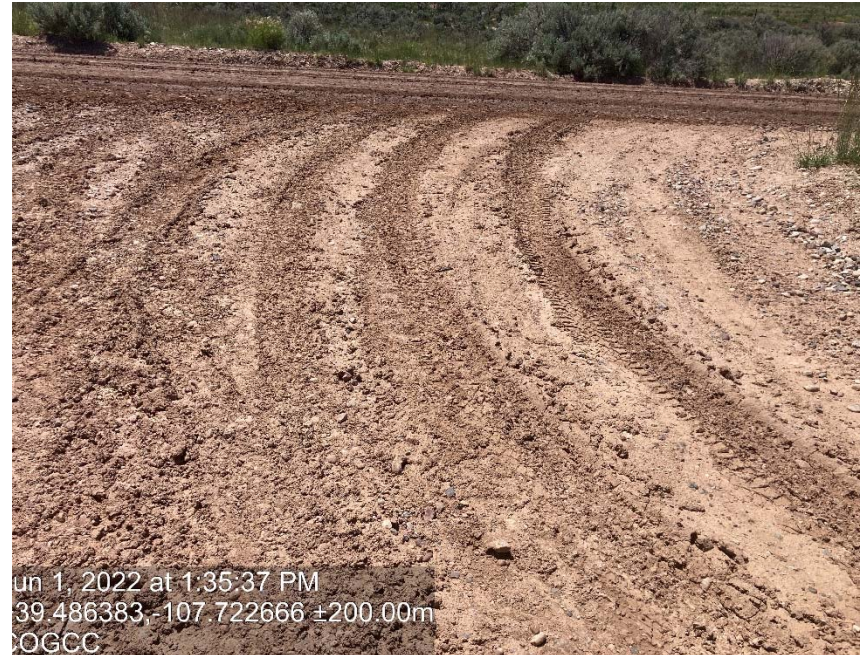
Lack of stabilization/ compaction
