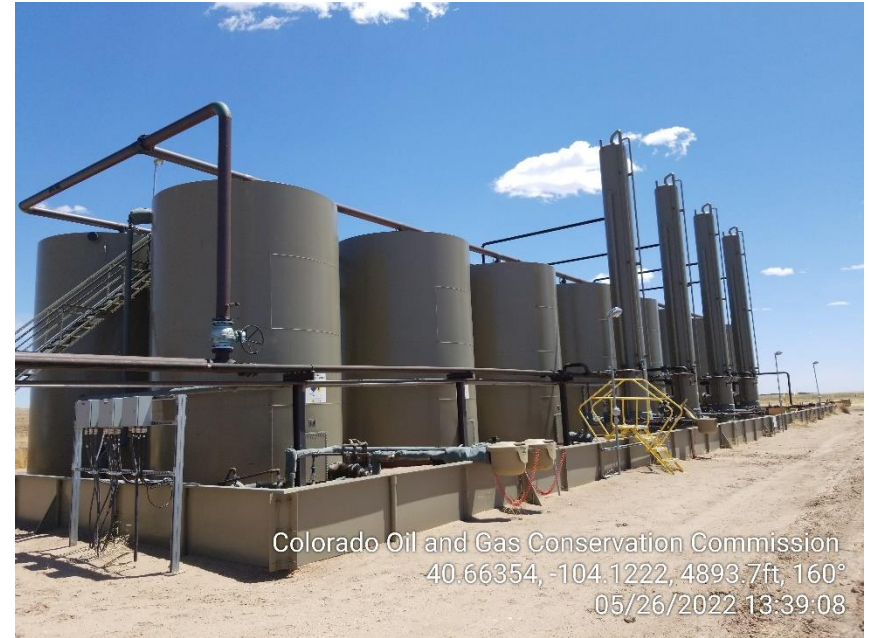
Photo 10 – Tank Battery
