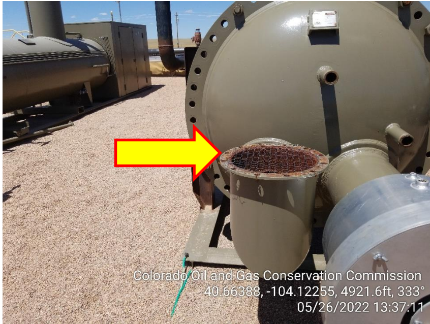
Photo 5 – Screen has been installed
