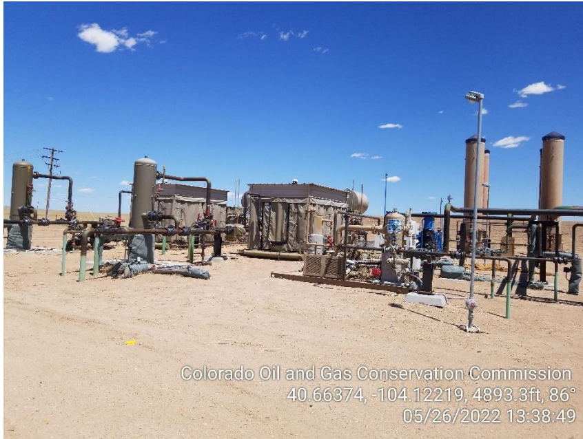
Photo 9 – Compressors, VRUs, and ECDs
