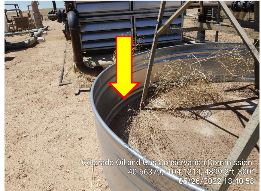
Photo 14 – Debris and Wildlife Netting in disrepair
