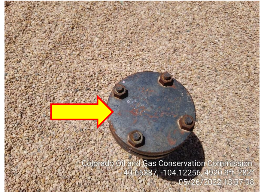
Photo 4 – Unmarked Riser at West Separators – Marking has faded No Longer visible
